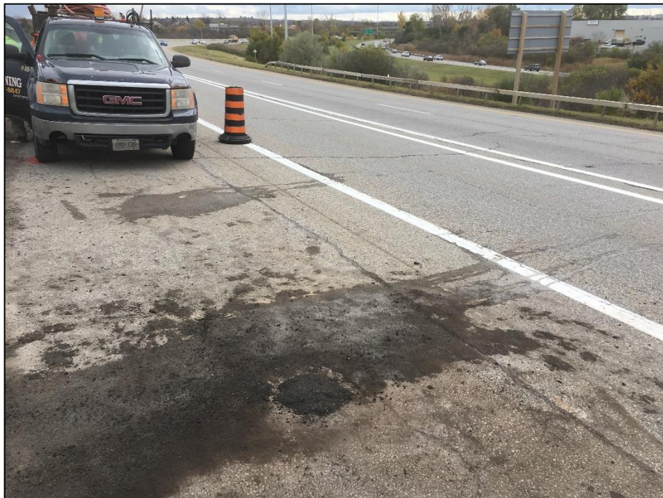
Photo 4. Borehole 17-02 upon completion of backfilling (2017-11-08).
