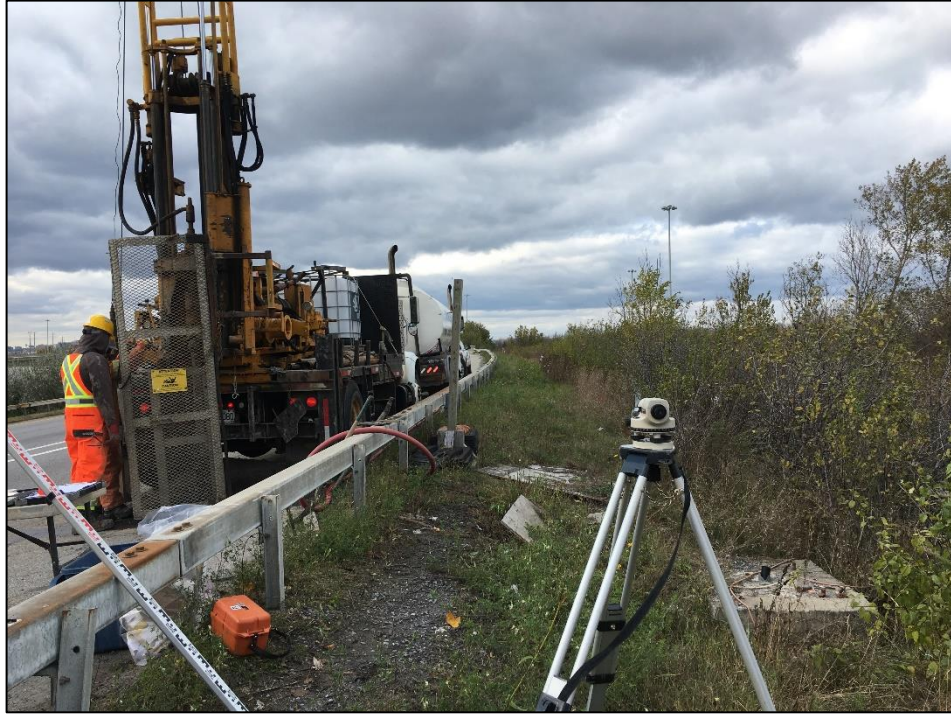
Photo 3. Drill rig set up on Borehole 17-02, looking northwest, old sign foundation visible to the right (2017-11-08).
