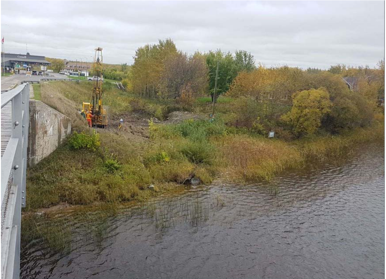
Photograph P3 – Drilling at the Location of Borehole 17-6, at the East Abutment of the Proposed Bridge on the Canadian side (October 03, 2017).
