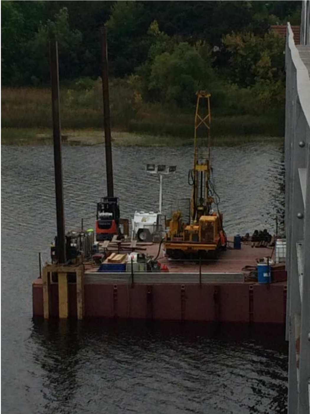
Photograph P2 – Drilling at the Location of Borehole 17-2, near Pier 2 of the Proposed Bridge on the US side (September 08, 2017).
