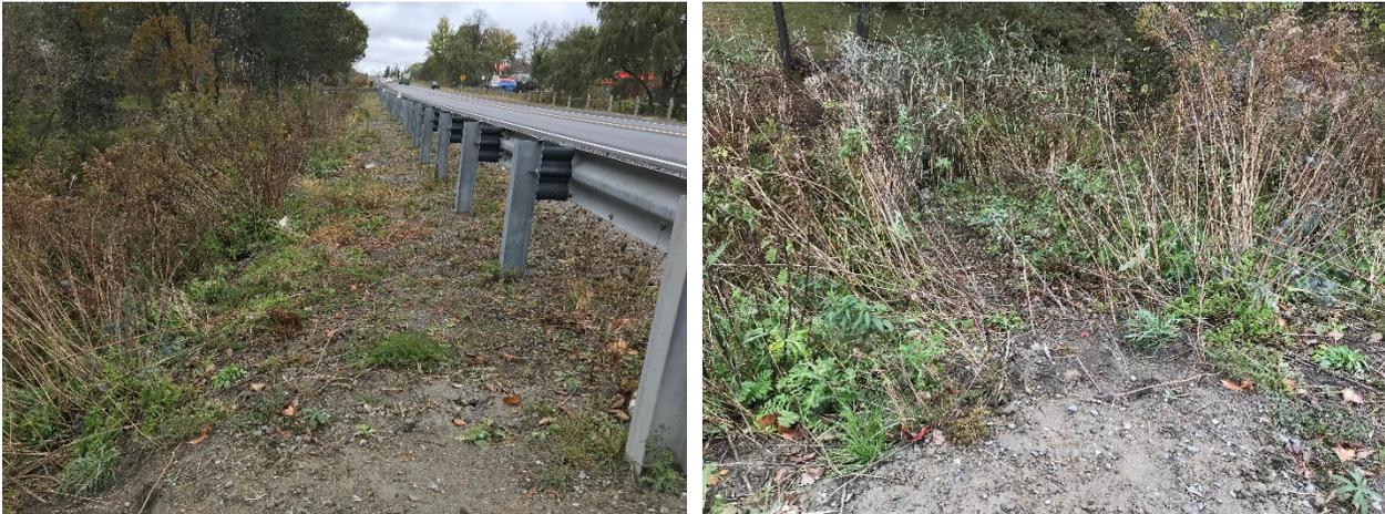
*Photograph 2: Surface erosion on west side of Highway 48*
