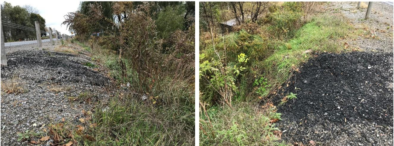
*Photograph 1: Surface erosion on east side of Highway 48*
