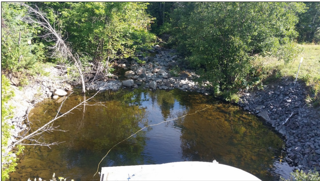
Photograph 4: Cobbles and boulders around and at the bottom of the scour pool as well as along the creek north of the scour pool (looking north/upstream from top of Highway 556)
