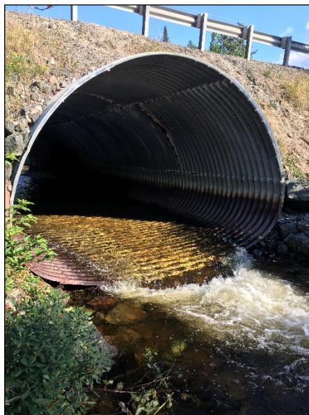
Photograph 2: Outlet of the northern SPCSPA culvert on the west side of Highway 532 (looking southeast)
