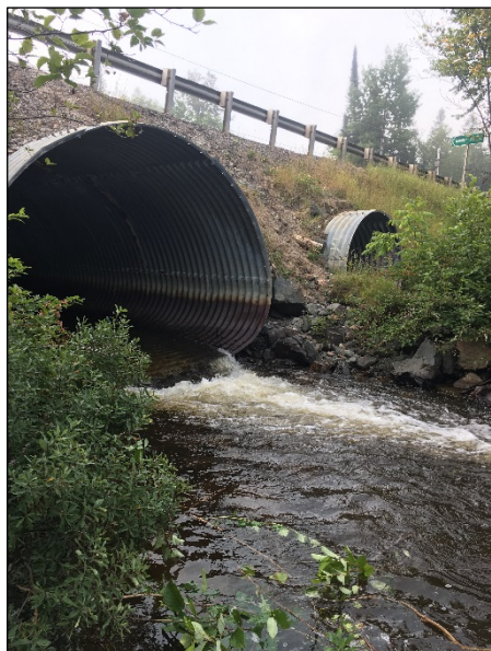
Photograph 1: Twin culverts at the Dam Creek site with Highway 532 above the culverts (looking southeast at the outlets)
