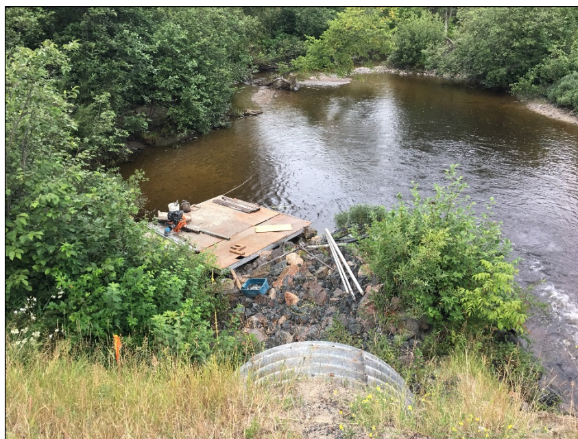
Photograph 4: Cobbles and boulders at the outlet of the southern SPCSP culvert (looking west from top of Highway 532)
