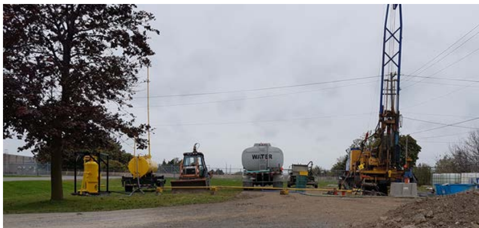
Photograph 6: Blow-out prevention system showing the degasser and venting stack (left) and drill (right)
