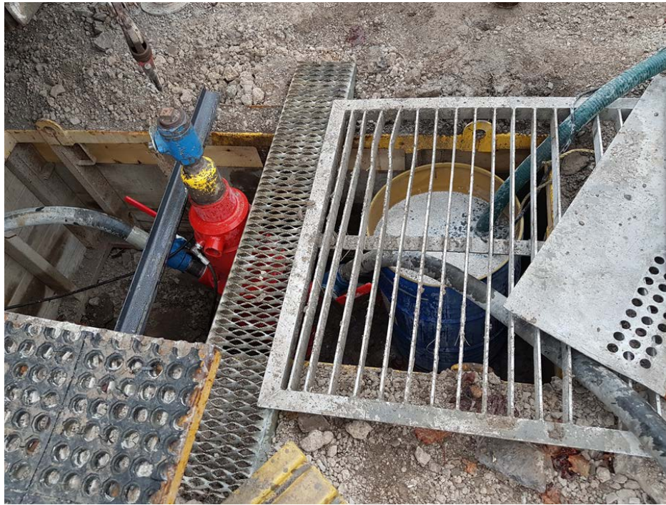
Photograph 7: Blow-out prevention system on the borehole
