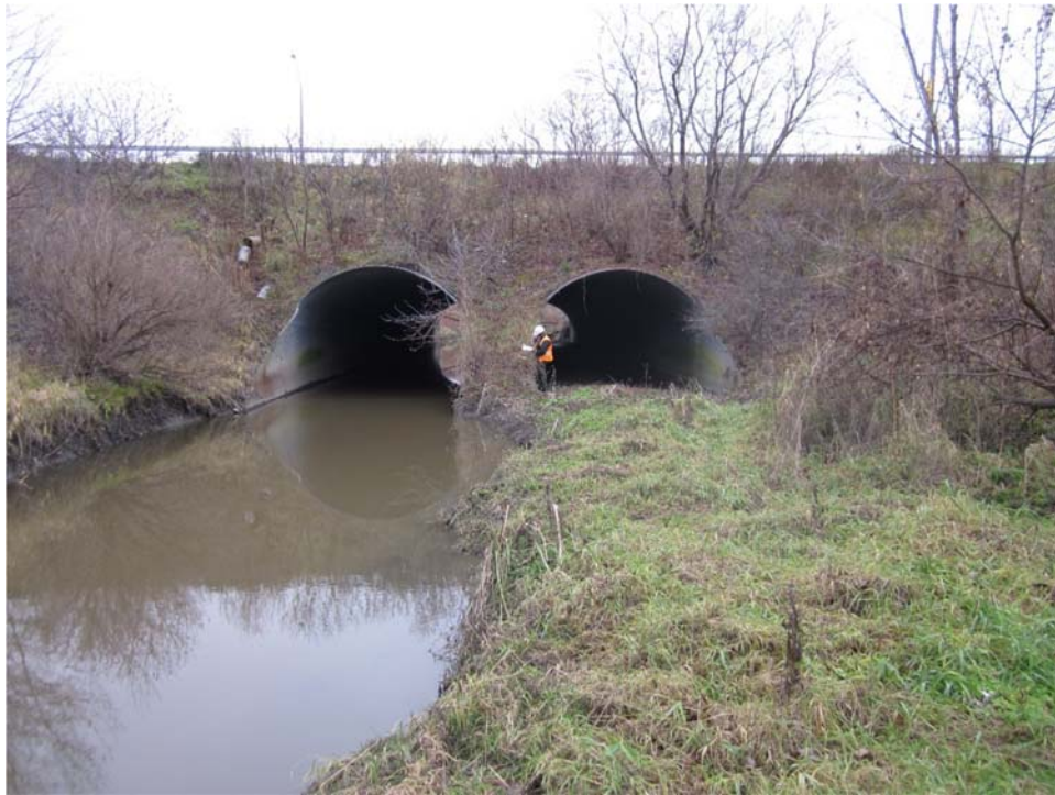
Photograph 1: Looking south towards culvert outlets
