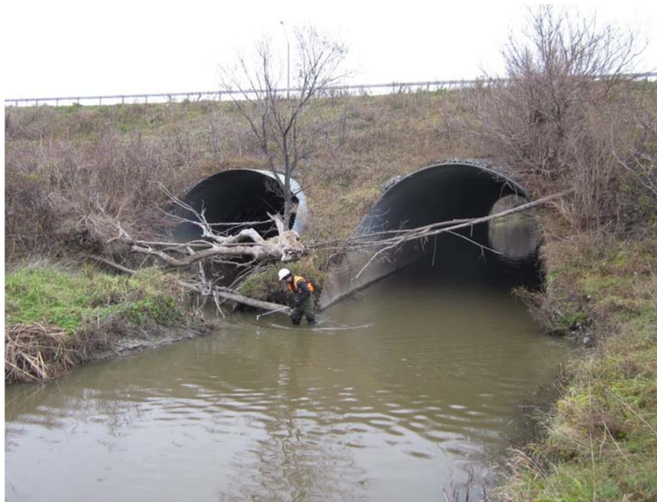
Photograph 2: Looking north towards culvert inlets
