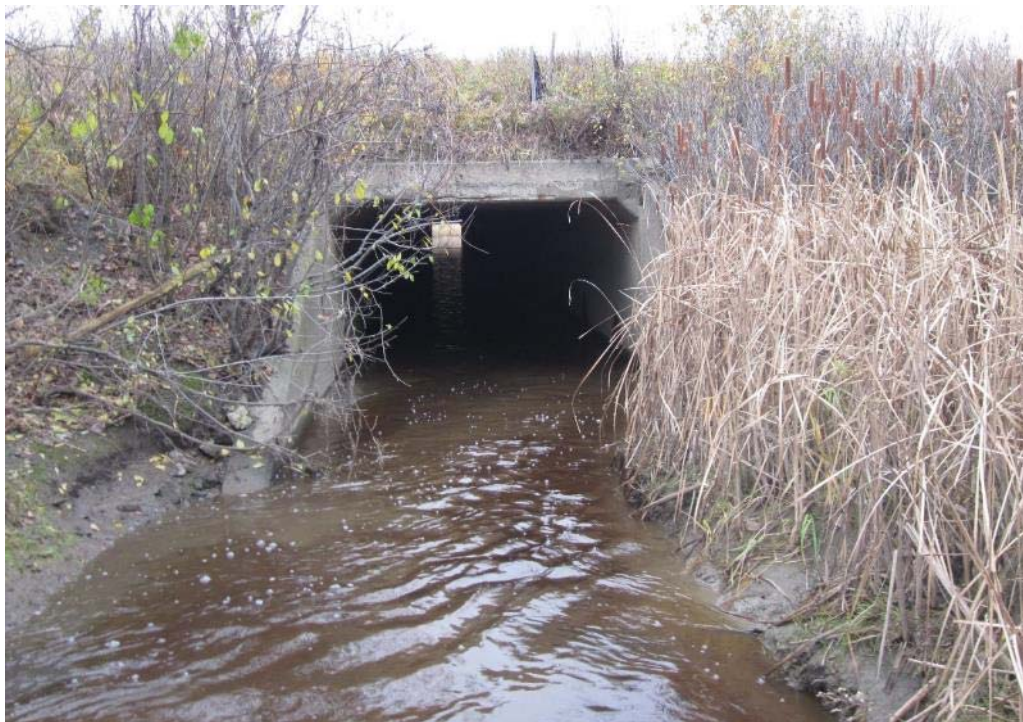
Photograph 2: Looking east towards culvert outlet
