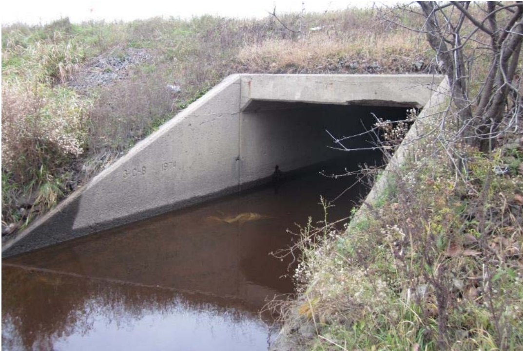
Photograph 1: Looking west towards culvert inlet
