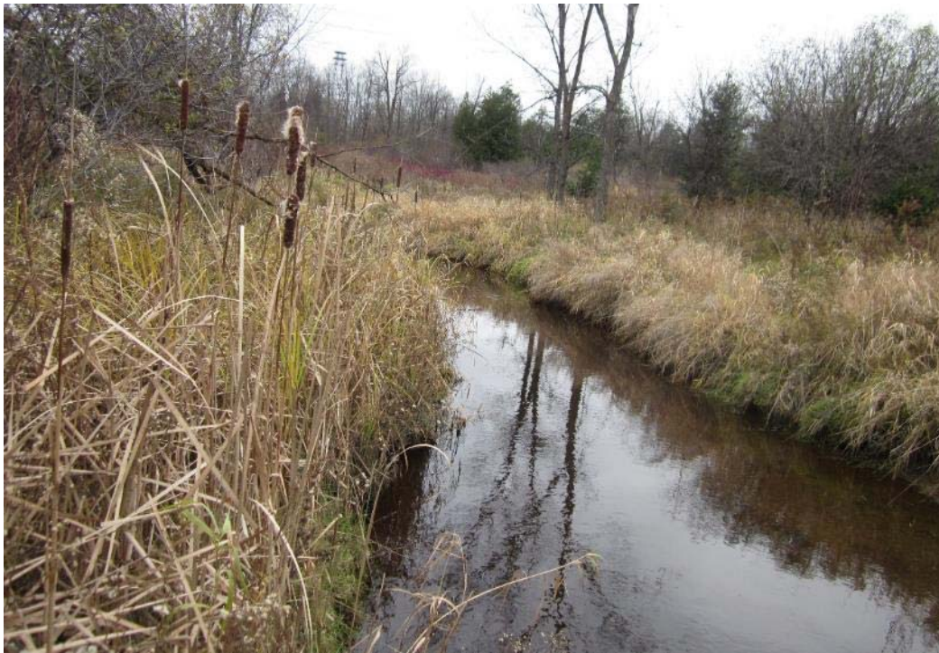
Photograph 3: Looking upstream from culvert inlet
