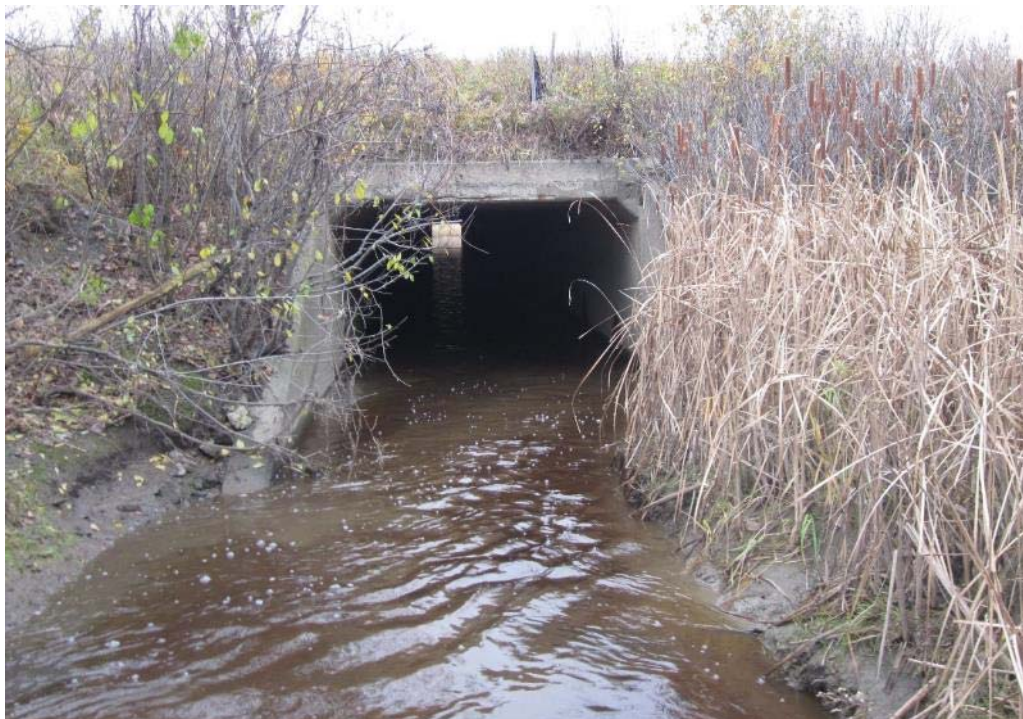
Photograph 2: Looking east towards culvert outlet
