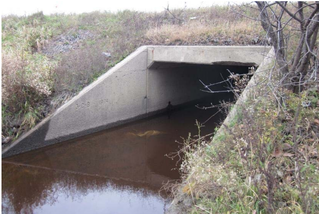
Photograph 1: Looking west towards culvert inlet
