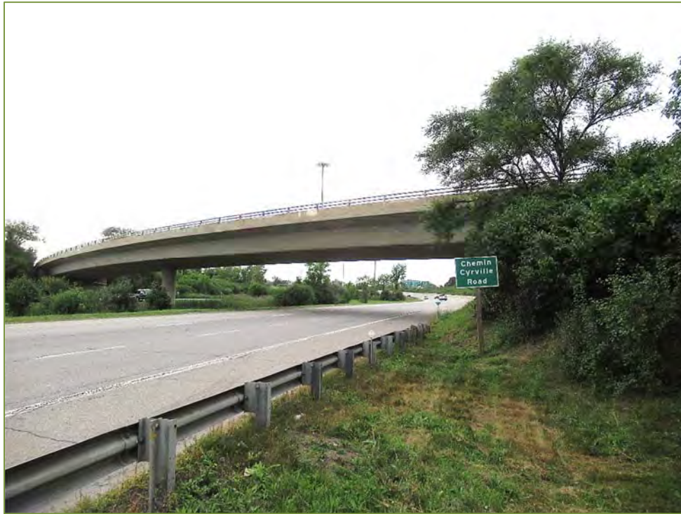
South Elevation - Looking towards HWY 417 WB
