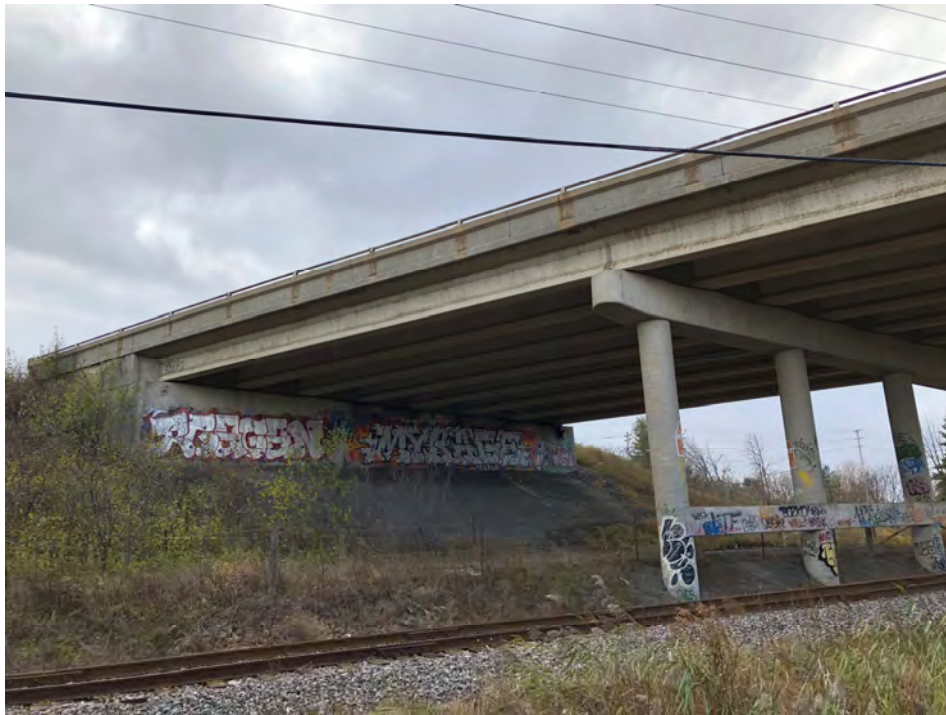
Photograph 2: South of west abutment of Site 3-302/1 (EBL), looking north (November 2018).
