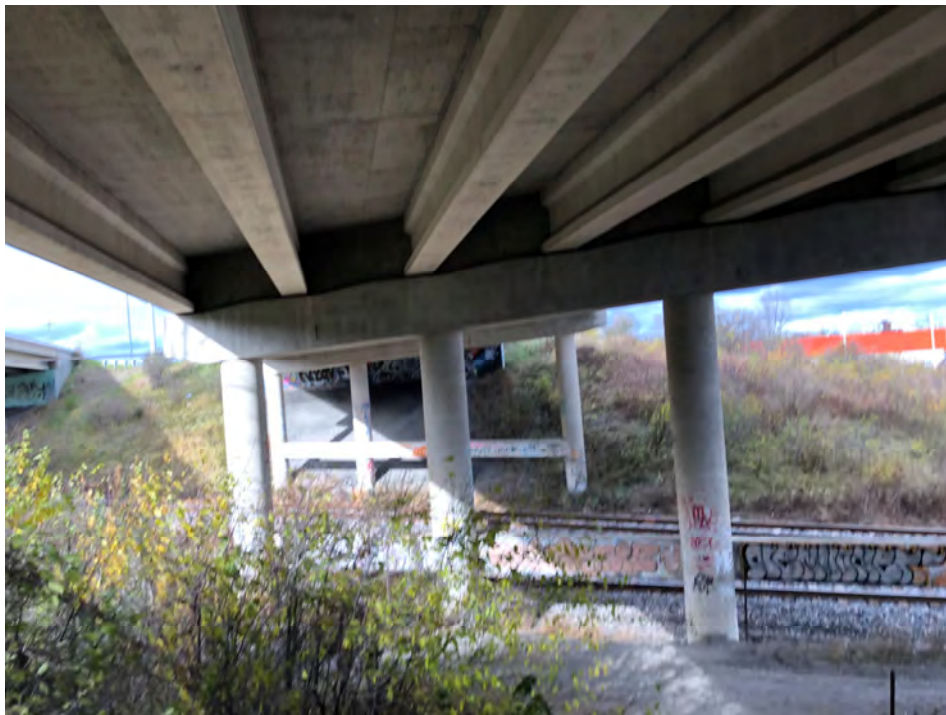
Photograph 4: West abutment and piers of Site 3-302/2 (WBL), looking northwest (November 2018).
