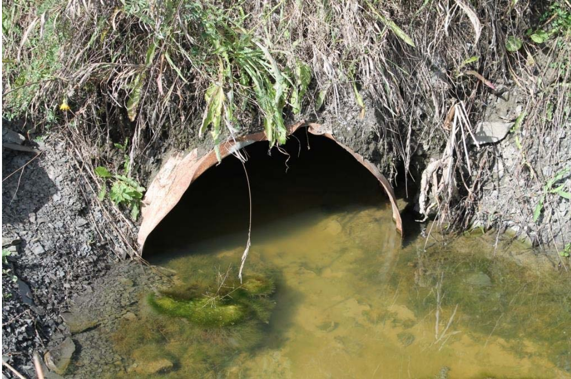
Photograph 1: Unnamed Creek Culvert (WBL), North inlet, looking south (provided by WSP).
