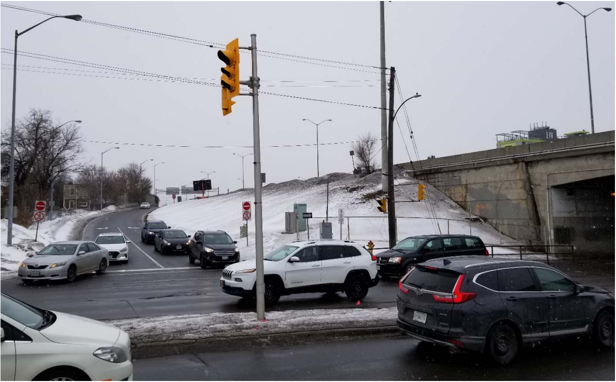
Photograph 5: Looking west towards the southwest embankment 2019-03-13
