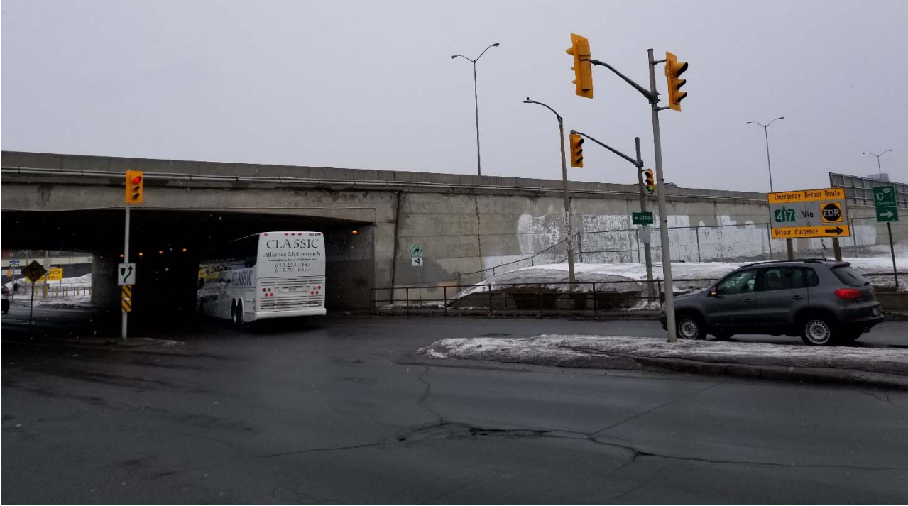
Photograph 6: Looking north towards the southeast retaining wall 2019-03-13
