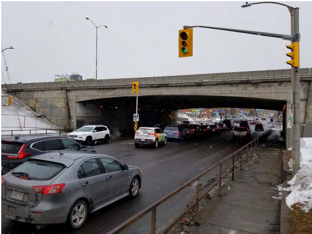
Photograph 1: Looking north along Bronson Avenue towards the Highway 417 Overpass at Bronson Avenue 2019-03-13
