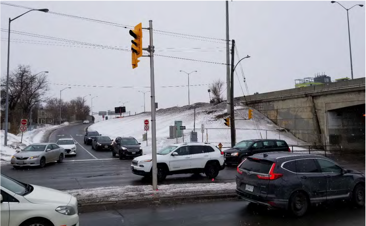
Photograph 5: Looking west towards the southwest embankment 2019-03-13
