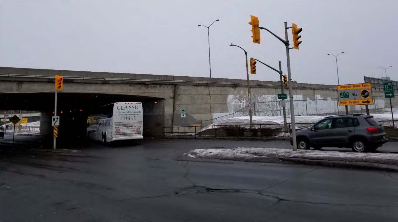
Photograph 6: Looking north towards the southeast retaining wall 2019-03-13
