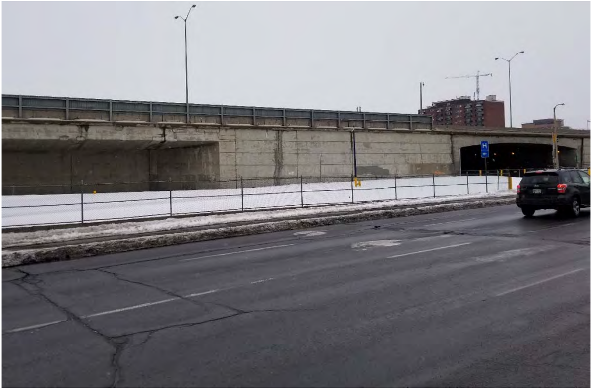
Photograph 3: Looking southwest towards existing northeast retaining wall east of east abutment 2019-03-13
