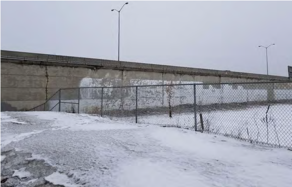
Photograph 4: Looking southwest towards existing northwest retaining wall west of west abutment 2019-03-13
