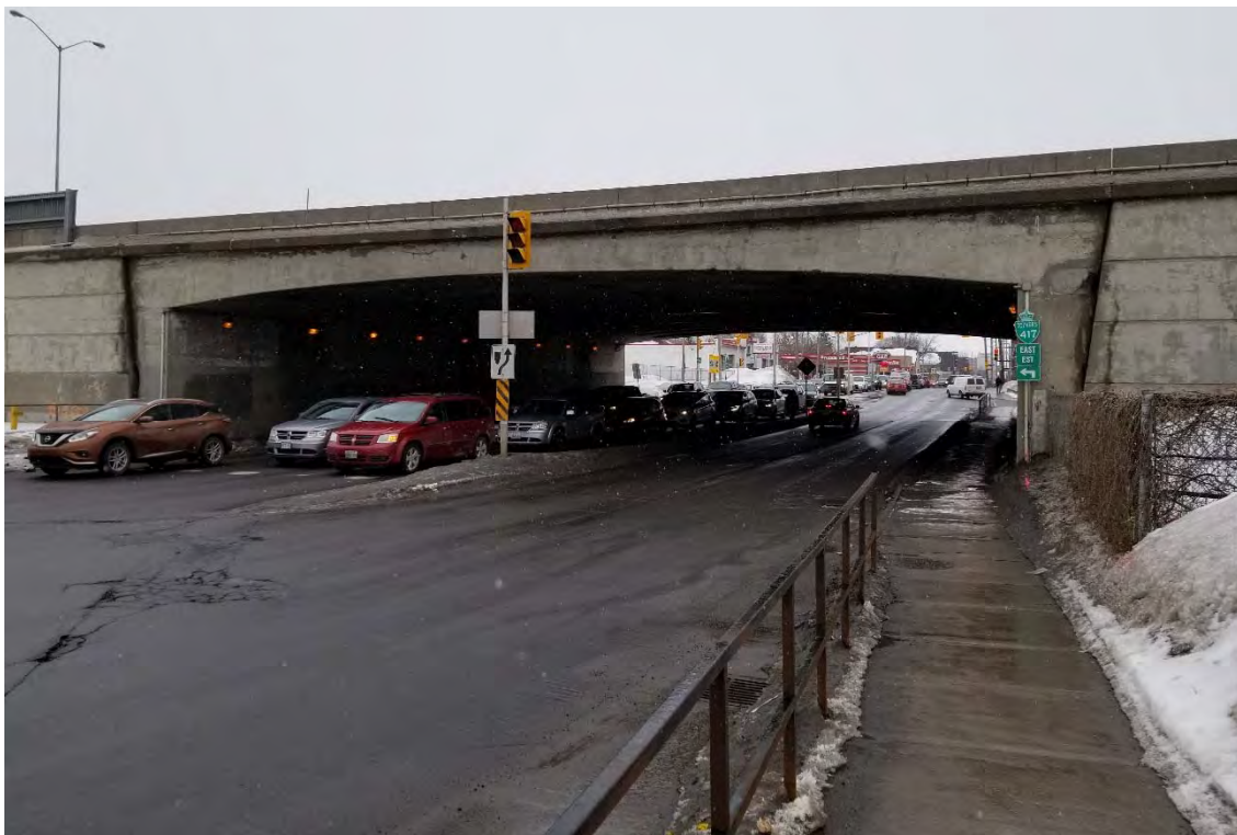
Photograph 2: Looking south towards the Highway 417 Overpass at Bronson Avenue 2019-03-13
