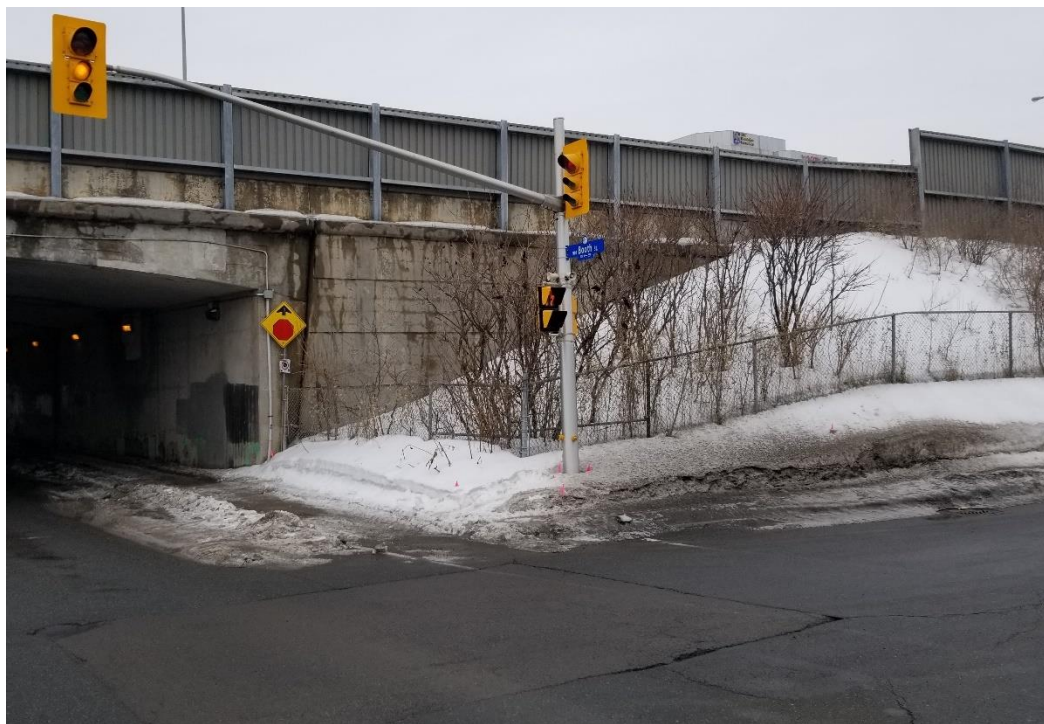
Photograph 4: Looking southwest towards the northwest embankment; 2019-03-13
