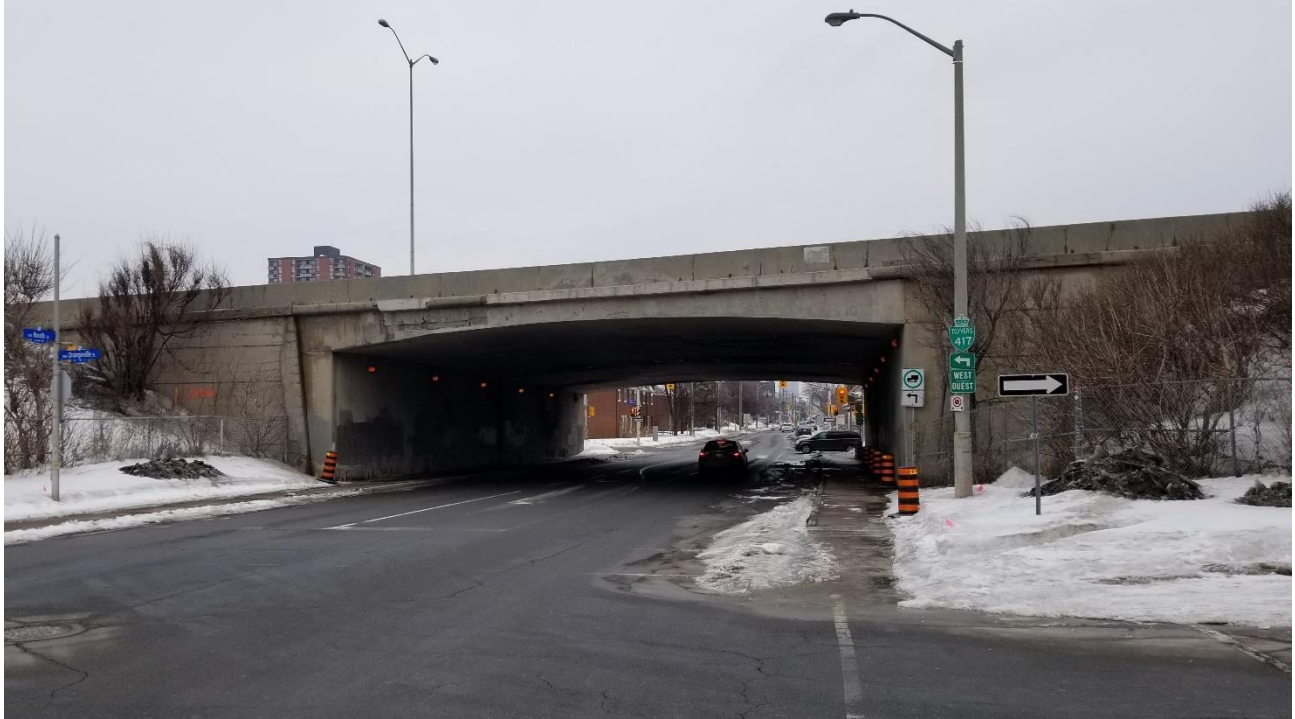
Photograph 1: Looking north along Booth Street towards the Highway 417 Overpass at Booth Street; 2019-03-13
