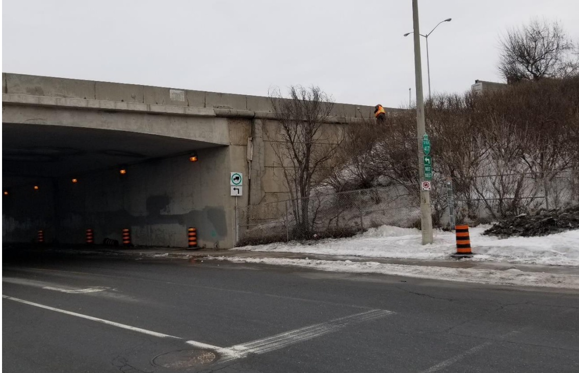
Photograph 5: Looking northeast towards the southeast embankment; 2019-03-13
