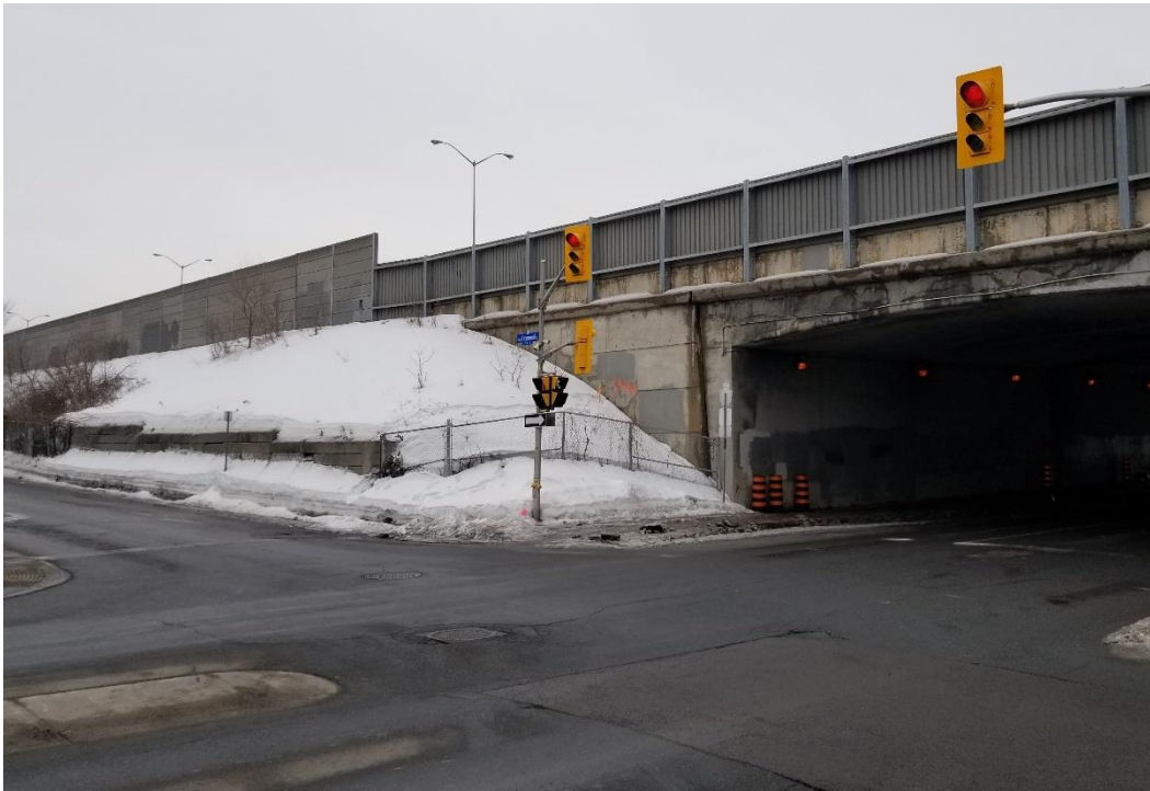
Photograph 3: Looking southeast towards the northeast embankment; 2019-03-13
