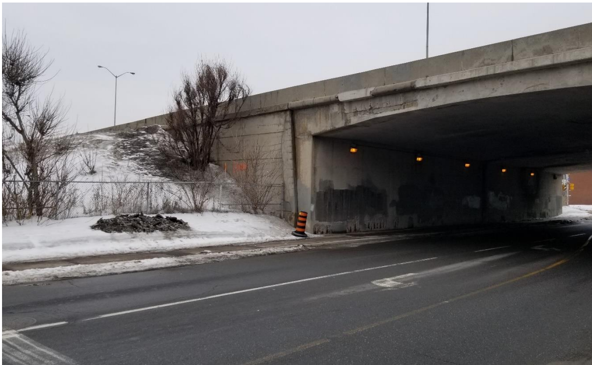
Photograph 6: Looking northwest towards the southwest embankment; 2019-03-13
