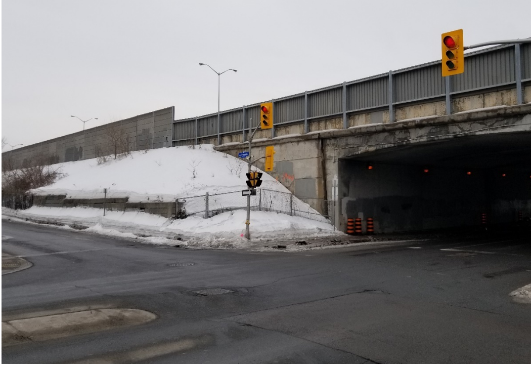
Photograph 3: Looking southeast towards the northeast embankment; 2019-03-13
