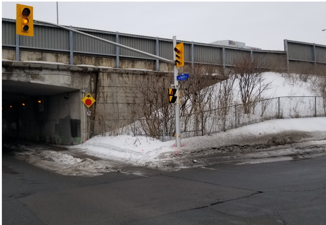
Photograph 4: Looking southwest towards the northwest embankment; 2019-03-13
