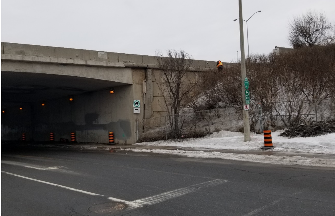
Photograph 5: Looking northeast towards the southeast embankment; 2019-03-13
