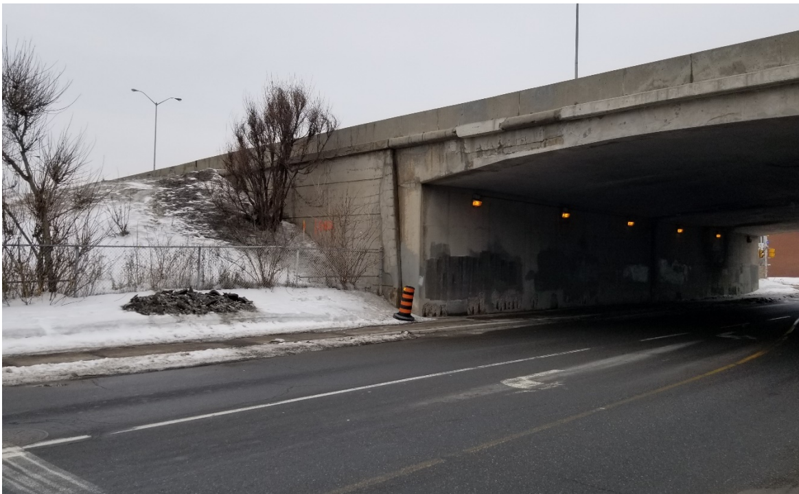
Photograph 6: Looking northwest towards the southwest embankment; 2019-03-13
