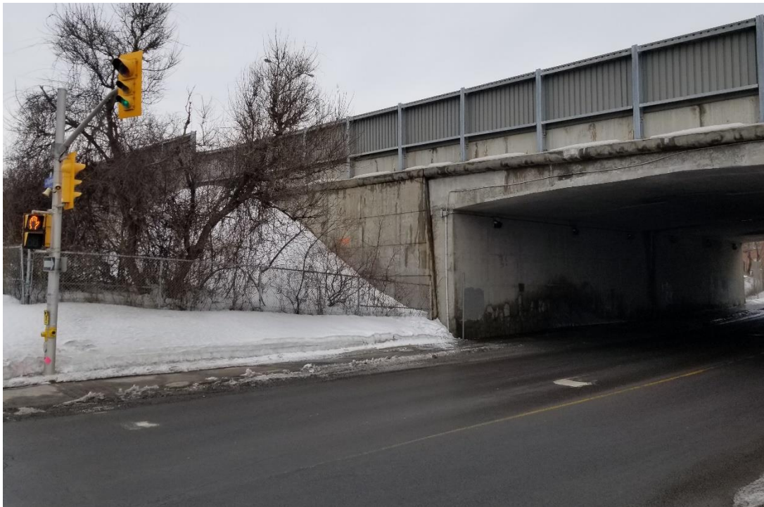
Photograph 3: Looking southeast towards the northeast embankment; 2019-03-13
