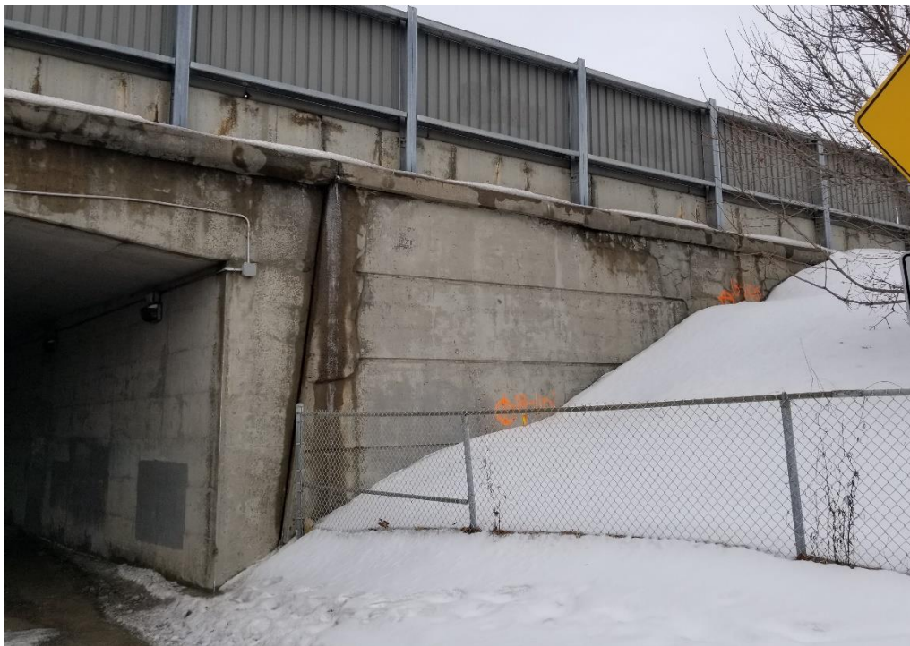
Photograph 4: Looking southwest towards the northwest embankment; 2019-03-13
