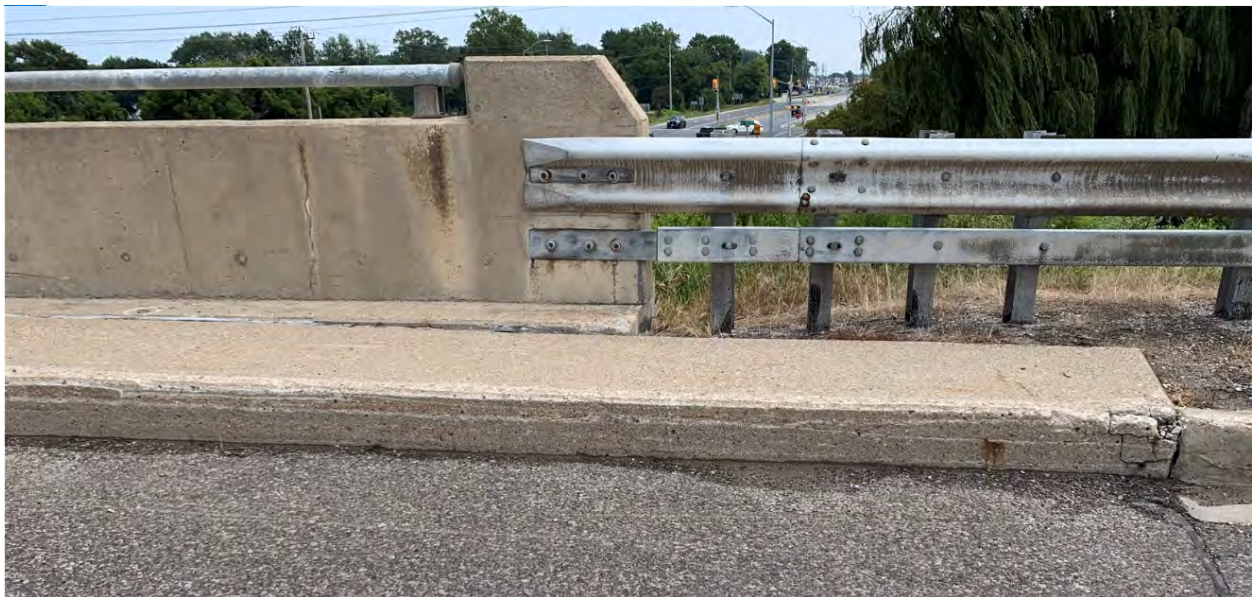
Photo 2: Settlement Between Approach Slab and Parapet Wall (East Bridge)
