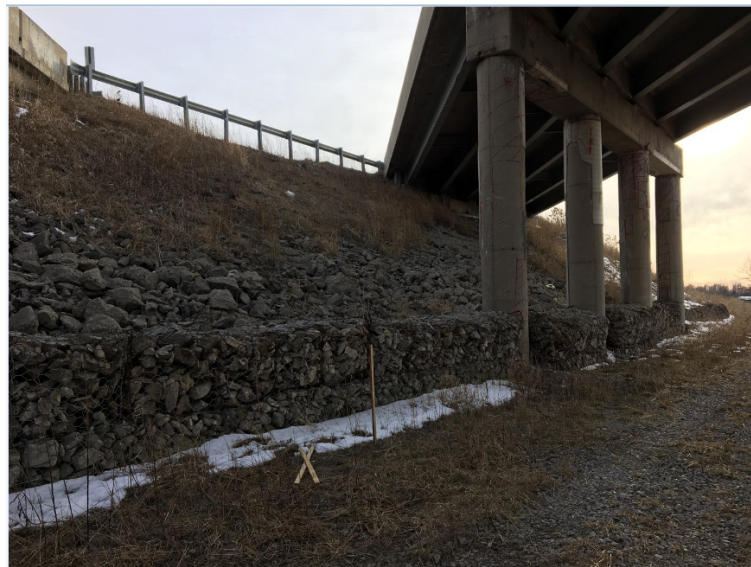
Photograph 3 – Gabion Basket Wall and Rockfill on Slope Face Below Bridge Abutments
