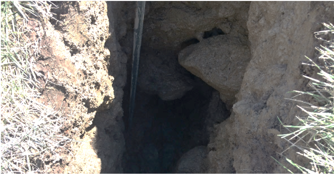
Photograph 2 – Boulders Within Hydro-Vac Excavation
