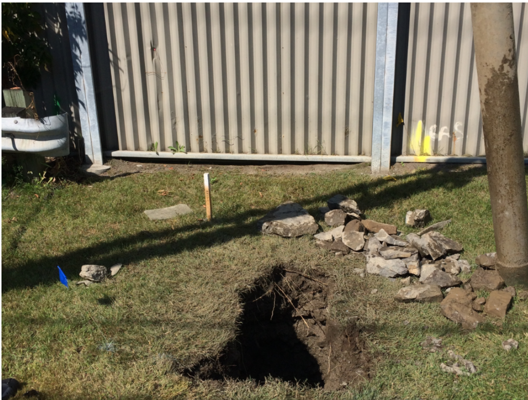
Photograph 1 – Cobbles and Boulders Excavated During Hydro-Vac Activities
