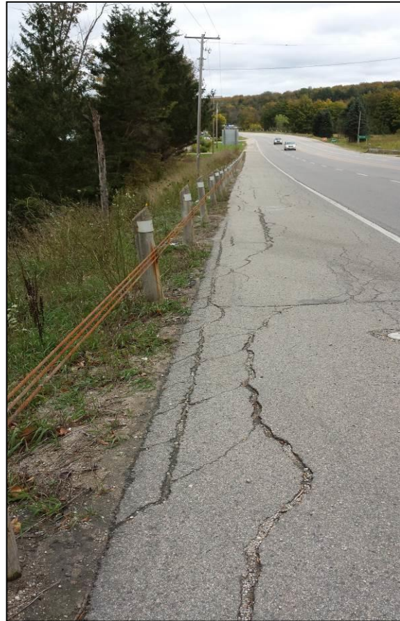
Photograph 9: Area 2 – Looking west from the location of the previous slope failure. Pavement distress and cracking along the westbound lane shoulder. (October 6, 2015)
