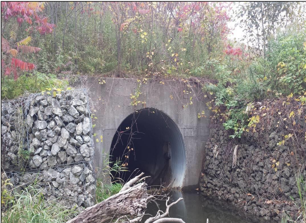
Photograph 2: Area 1 - Looking north at the location of existing CSP culvert. The culvert inlet and rip-rap protection is visible. (October 6, 2015)
