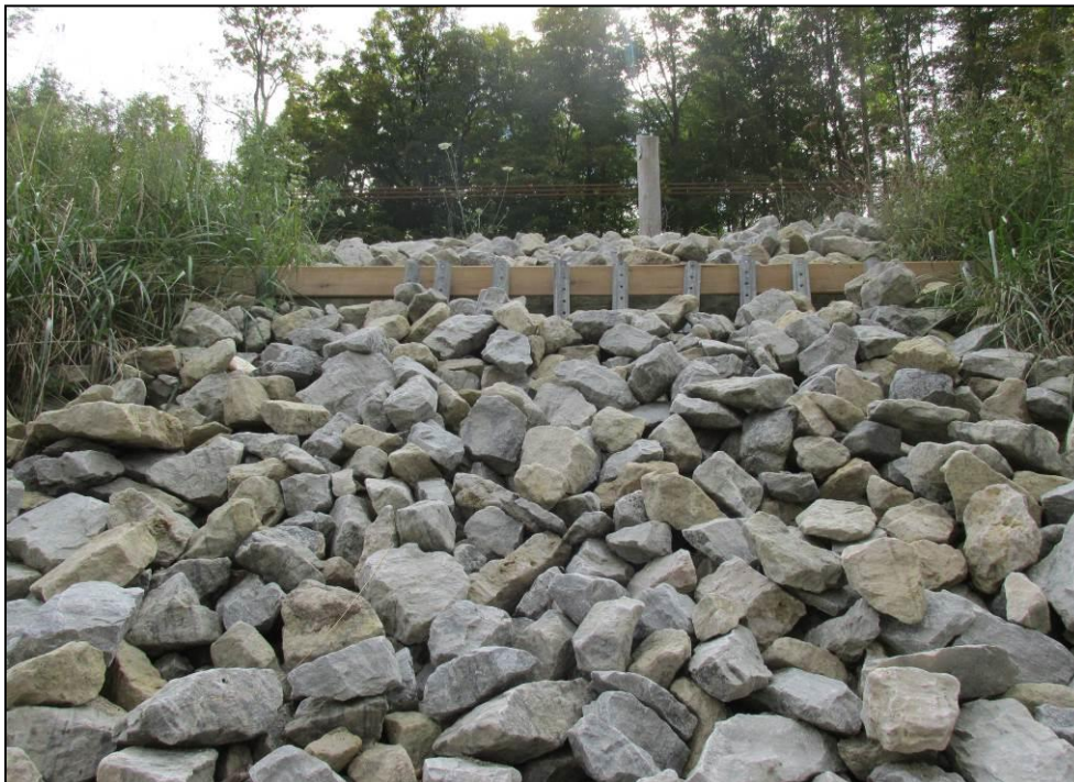
Photograph 7: Area 2 - Looking up from toe of the slope. Previous remedial measure for the surficial slope instability and partial timber cribbing is visible (October 6, 2015)
