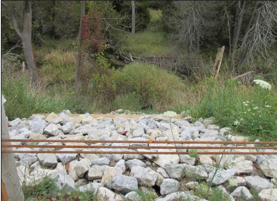
Photograph 6: Area 2 - Looking down from top of the slope. Previous remedial measure for the surficial slope instability. (October 6, 2015)
