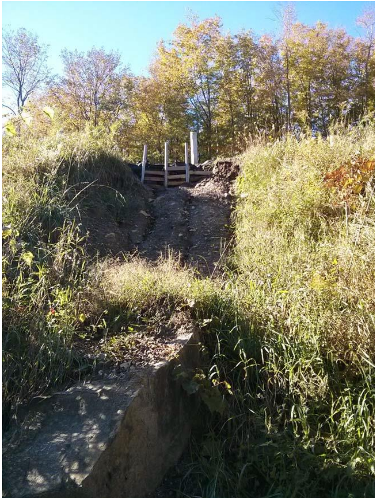
Photo 4 (from previous report): Looking Southward (toward Highway) from north toe of slope showing erosion gullies and soil deposition along slope failure on north side of highway. (2013)
