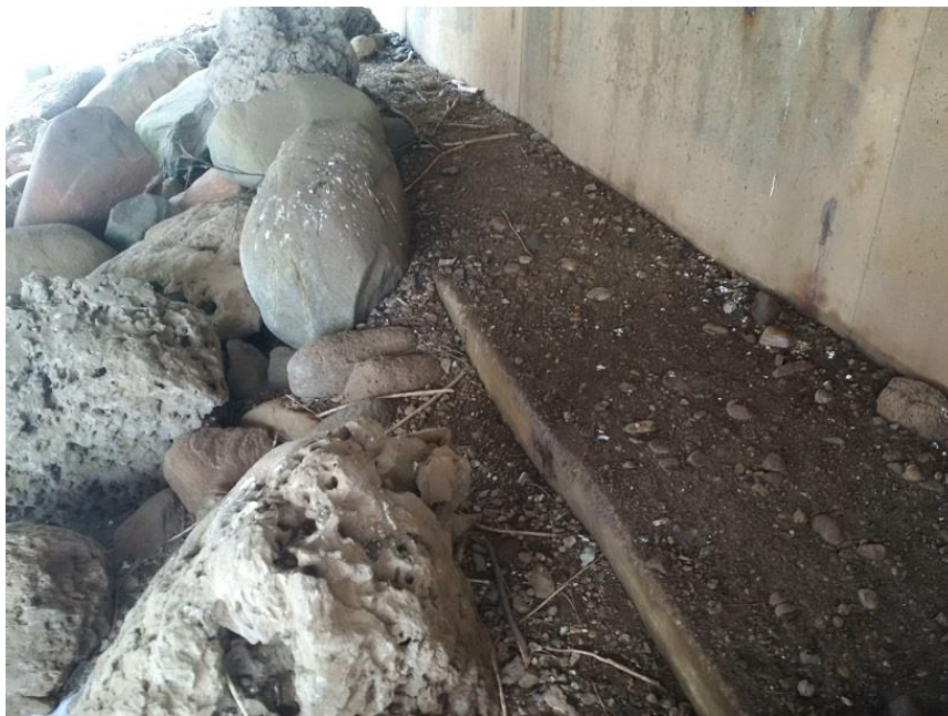
Photograph 8: Partially exposed pile cap at east abutment.
