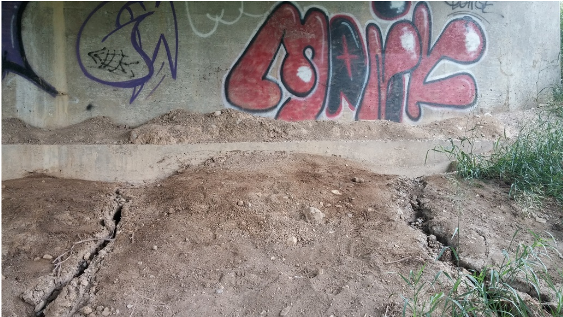
Photograph 3: North abutment. Note exposed pile cap as well as erosion and settlement.
