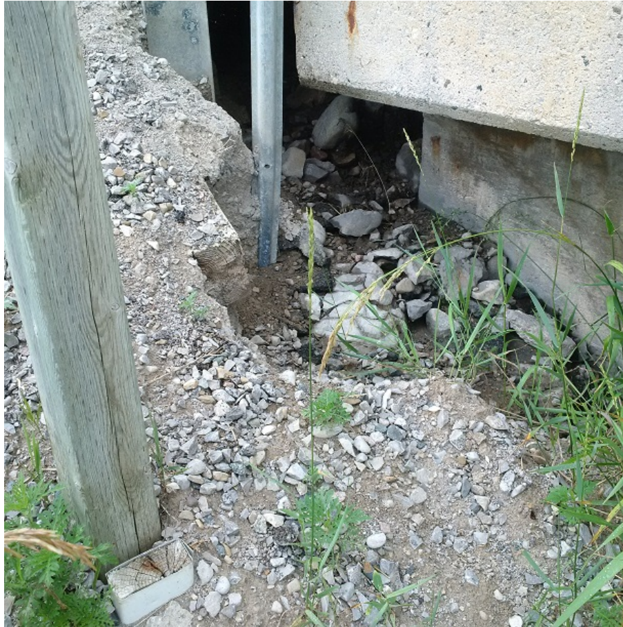
Photograph 9: North abutment on west side. Note erosion around abutment and under approach slab.
