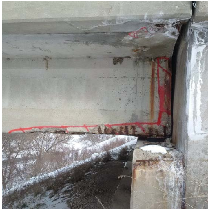
Photograph 6: South abutment at west end. Note apparent rotation, spalled concrete and exposed rebar.
