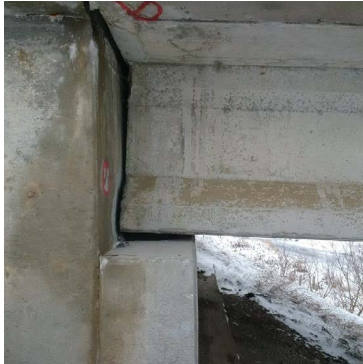
Photograph 5: South abutment at east end. Note apparent rotation.
