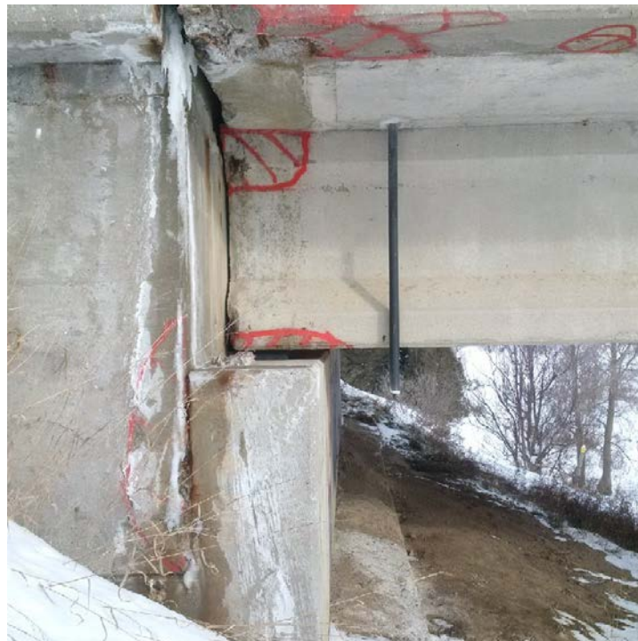
Photograph 8: North abutment at west end. Note apparent rotation, spalled concrete and exposed rebar.
