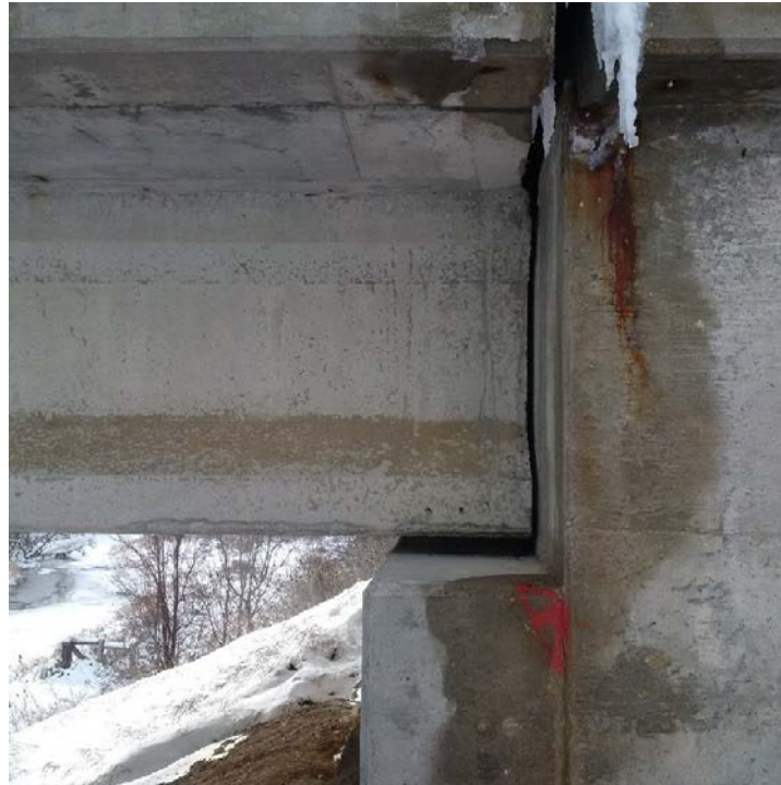
Photograph 7: North abutment at east end. Note spalled concrete and exposed rebar.
