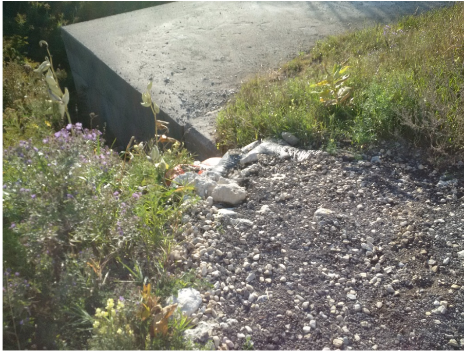
Photograph 5: East side (outlet) of Culvert Site 4-174/C. Photo taken in October 2016. Note sand bags and fill placed along north elevation.
