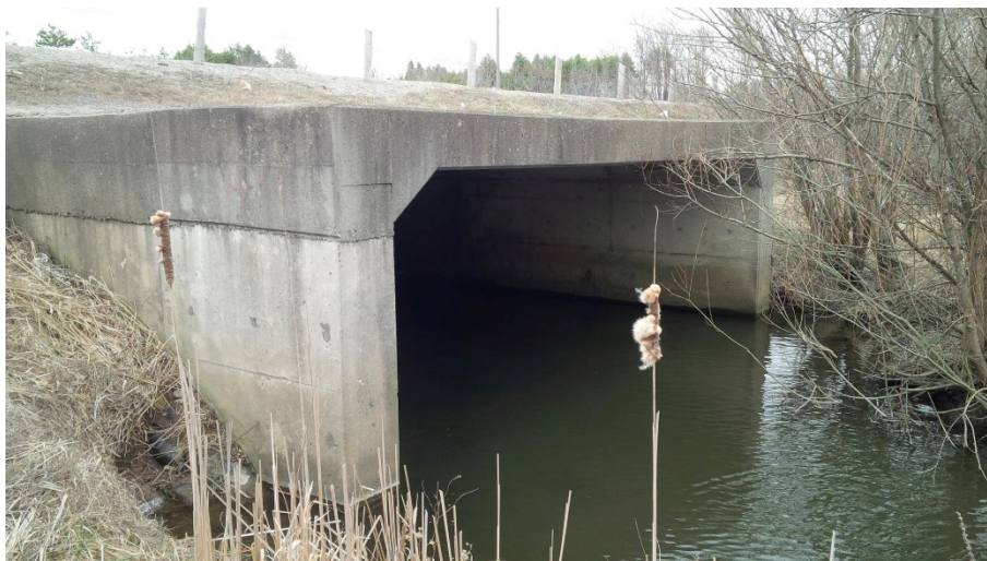
Photograph 2: West elevation (inlet) of Culvert Site 4-174/C. Note erosion at north elevation.
