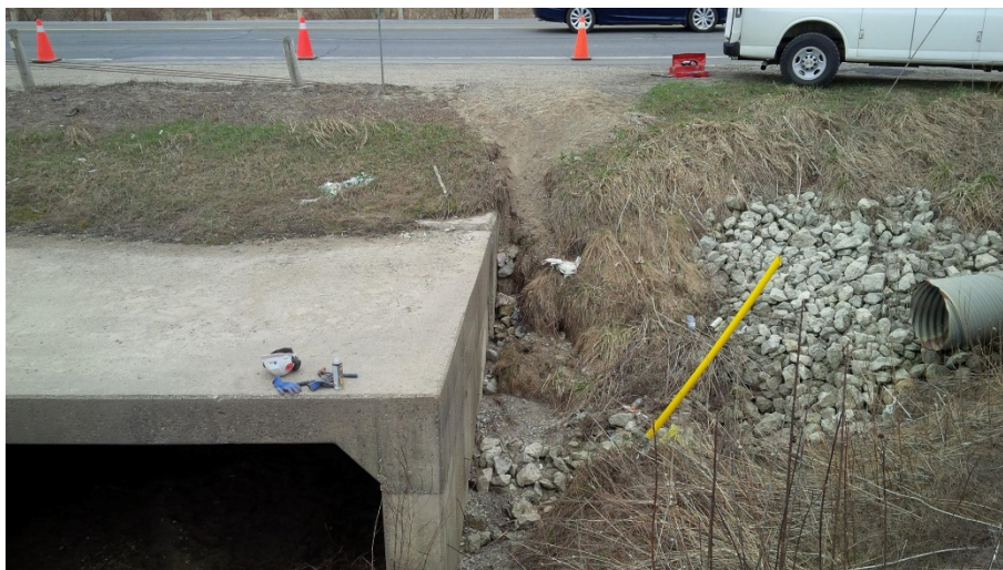
Photograph 4: East side (outlet) of Culvert Site 4-174/C. Photo taken in April 2016. Note erosion along north elevation.
