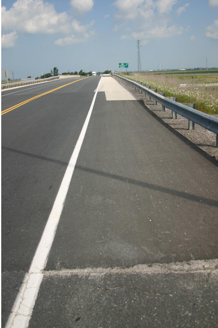
Looking north at patch above 36 inch diameter concrete culvert along Highway 77 (August 17, 2015)
