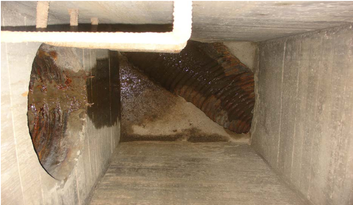
Photograph 8: View inside the MH # 19. Two pipes are connected to the manhole. The west wall inlet pipe originates from MH # 18 and the bottom pipe runs from the highway toward the Don River. (July 2015)
