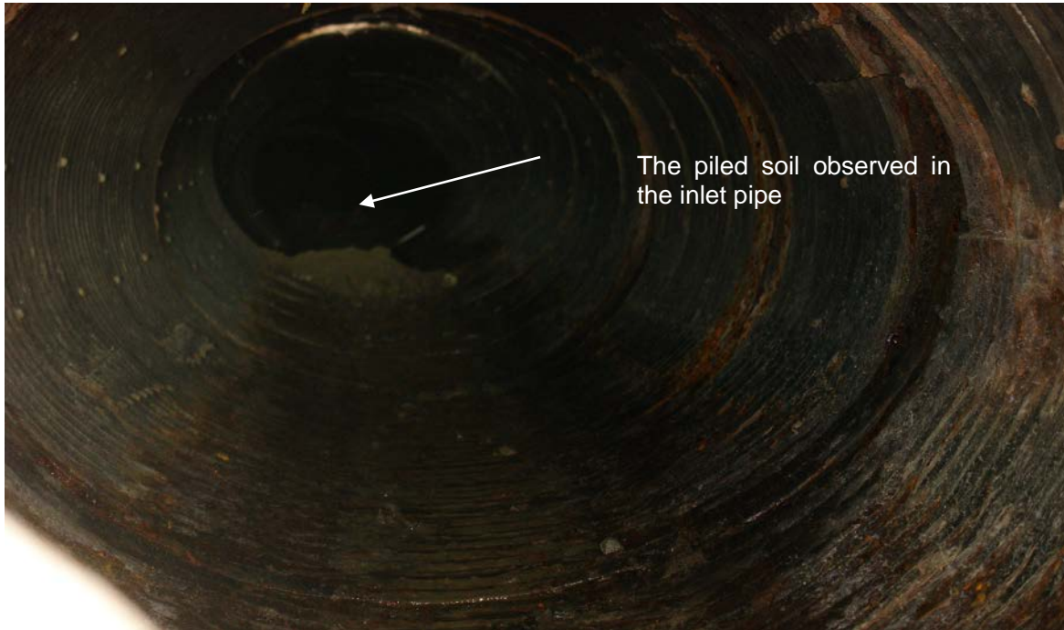
Photograph 9: The inlet pipe to MH # 19 inspected visually. A soil pile was observed in the inlet pipe and a small amount of water flow. (July 2015)
