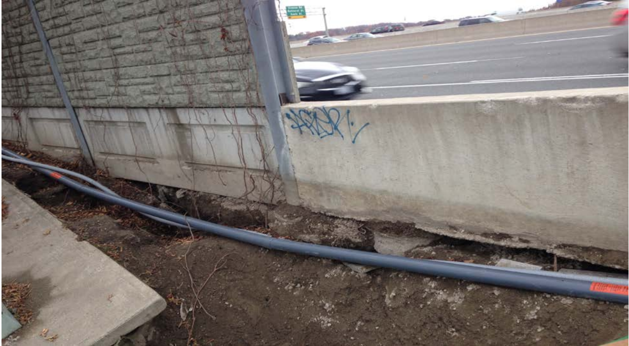
Photograph 1: Looking at the sinkhole toward Hwy 401. The fill material under the barrier wall and highway pavement caved into the sinkhole. (November 2014)
