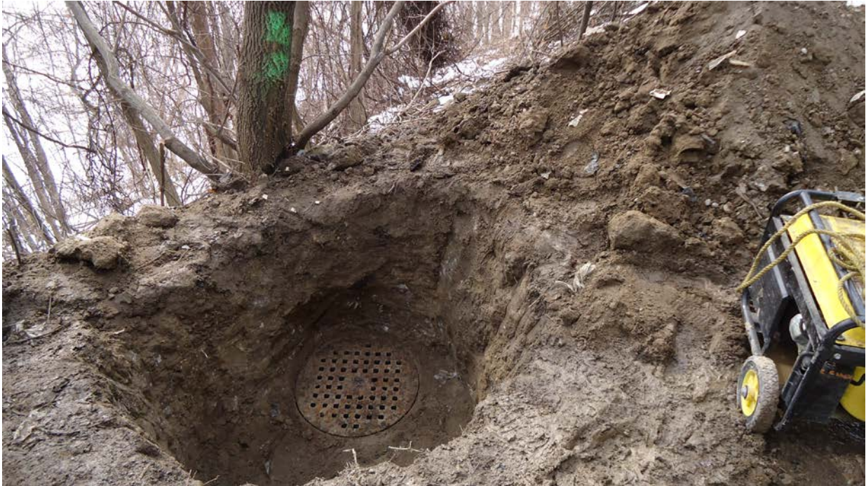
Photograph 3: Manhole # 18 was uncovered under about 1.5 m of frozen fill layer. (March 2015)
