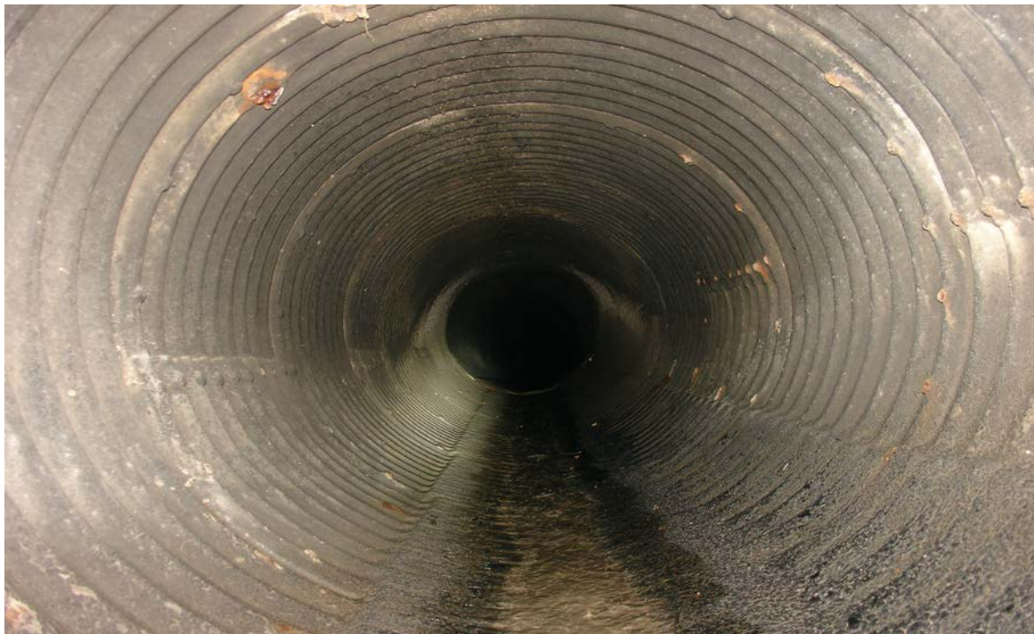
Photograph 10: View inside the pipe connected to the bottom level of MH # 19 running toward north to the highway. A small water flow was noted. (July 2015)
