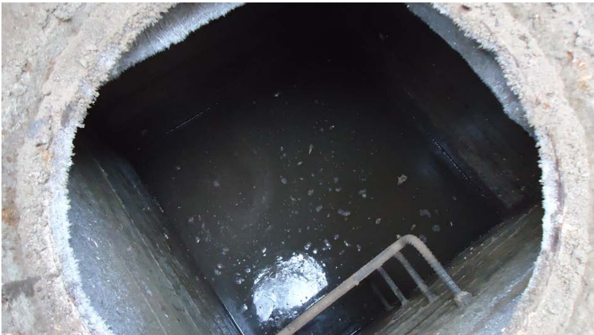
Photograph 4: The manhole #18 was full of water and the inlet and outlet pipes were placed under water suggesting a blockage downstream. (March 2015)
