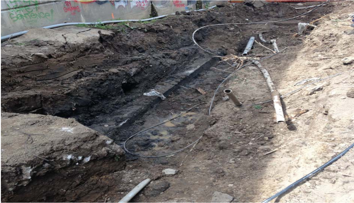
Photograph 7: The MH # 19 was found under about 1 m of fill. Several utility cables pass adjacent to the manhole. (July 2015)
