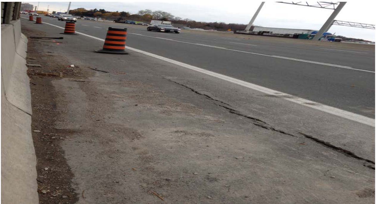
Photograph 2: Several cracks were observed during a site visit on the right shoulder of collector lanes likely resulted by loss of material under the pavement. (November 2014)
