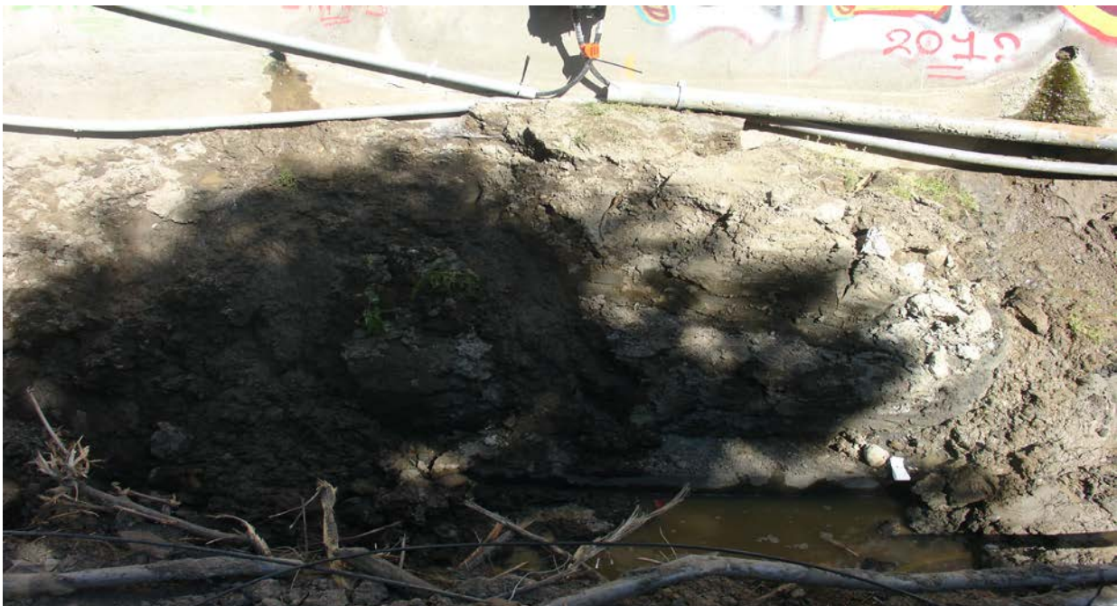
Photograph 6: Showing the weeping hole source of water possibly from highway catch basins. Water collects in the MH # 19 surrounding area. (July 2015)
