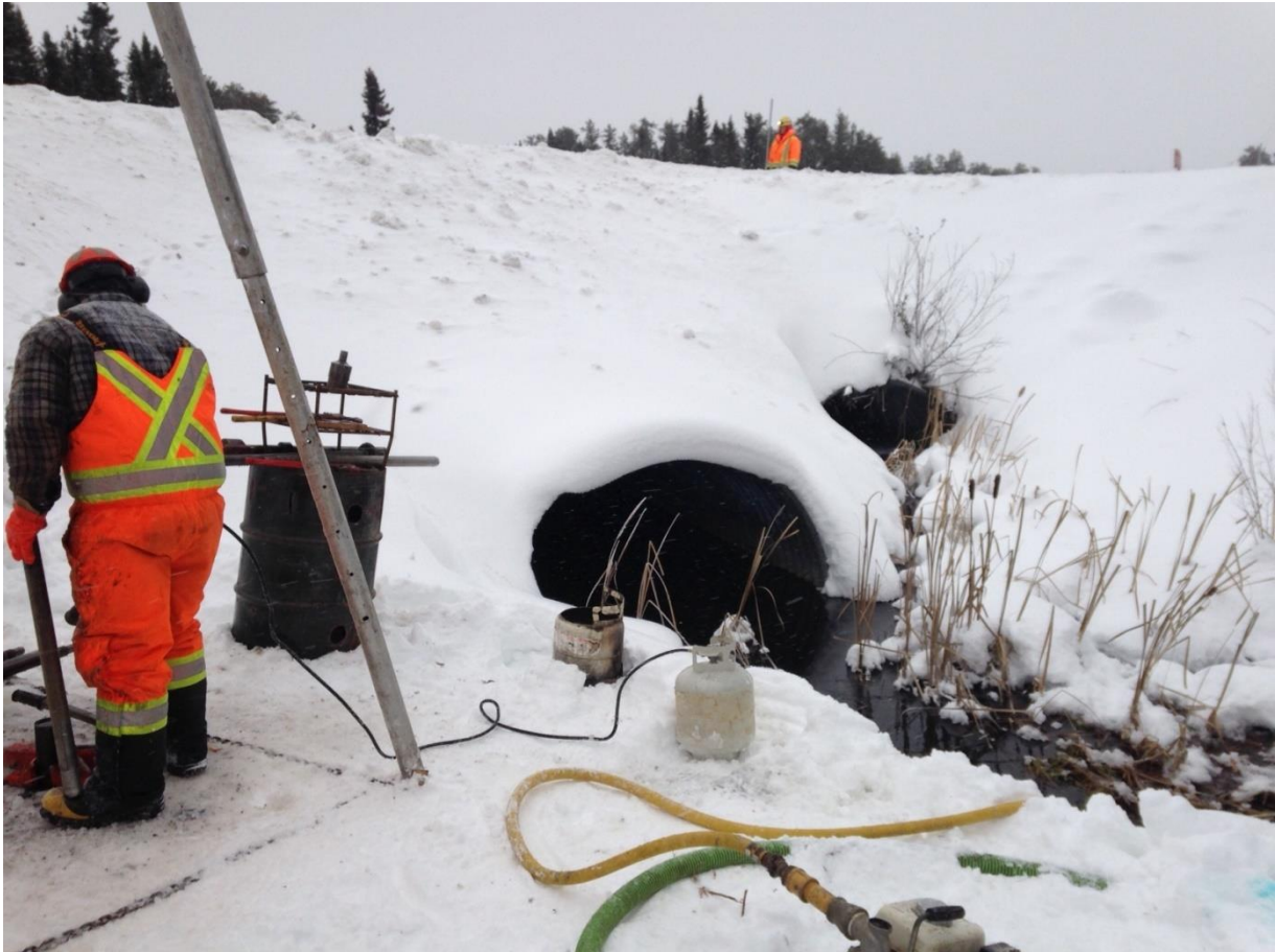
Photograph P4: Looking west from toe of Highway 129 embankment. Borehole TC4 was drilled at northeast of the culvert inlet. The inlet of the existing twin culvert is visible. (January 17, 2015)
