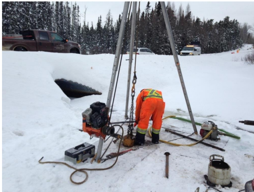
Photograph V4: Looking north to Vincent Creek outlet. The slope was covered with ice and snow at the time of the investigation. The borehole VC-4 was advanced using a manual method (tripod). (January, 2015)
