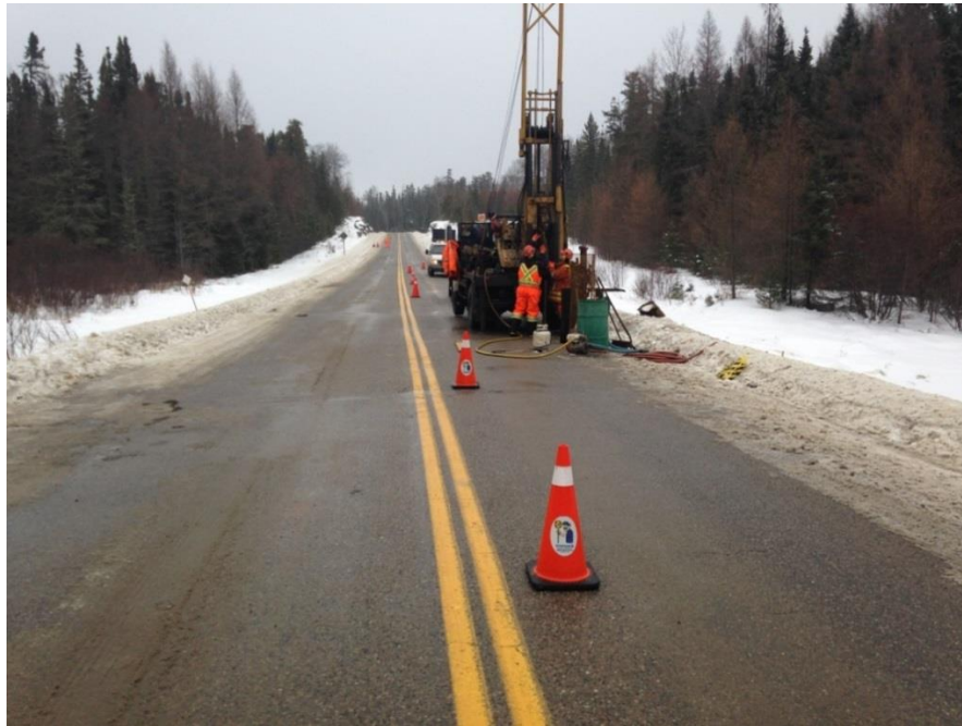
Photograph V3: Looking north from center of Highway 129. Borehole VC-3 advanced using a truck mounted drill rig at this location. (December, 2014)
