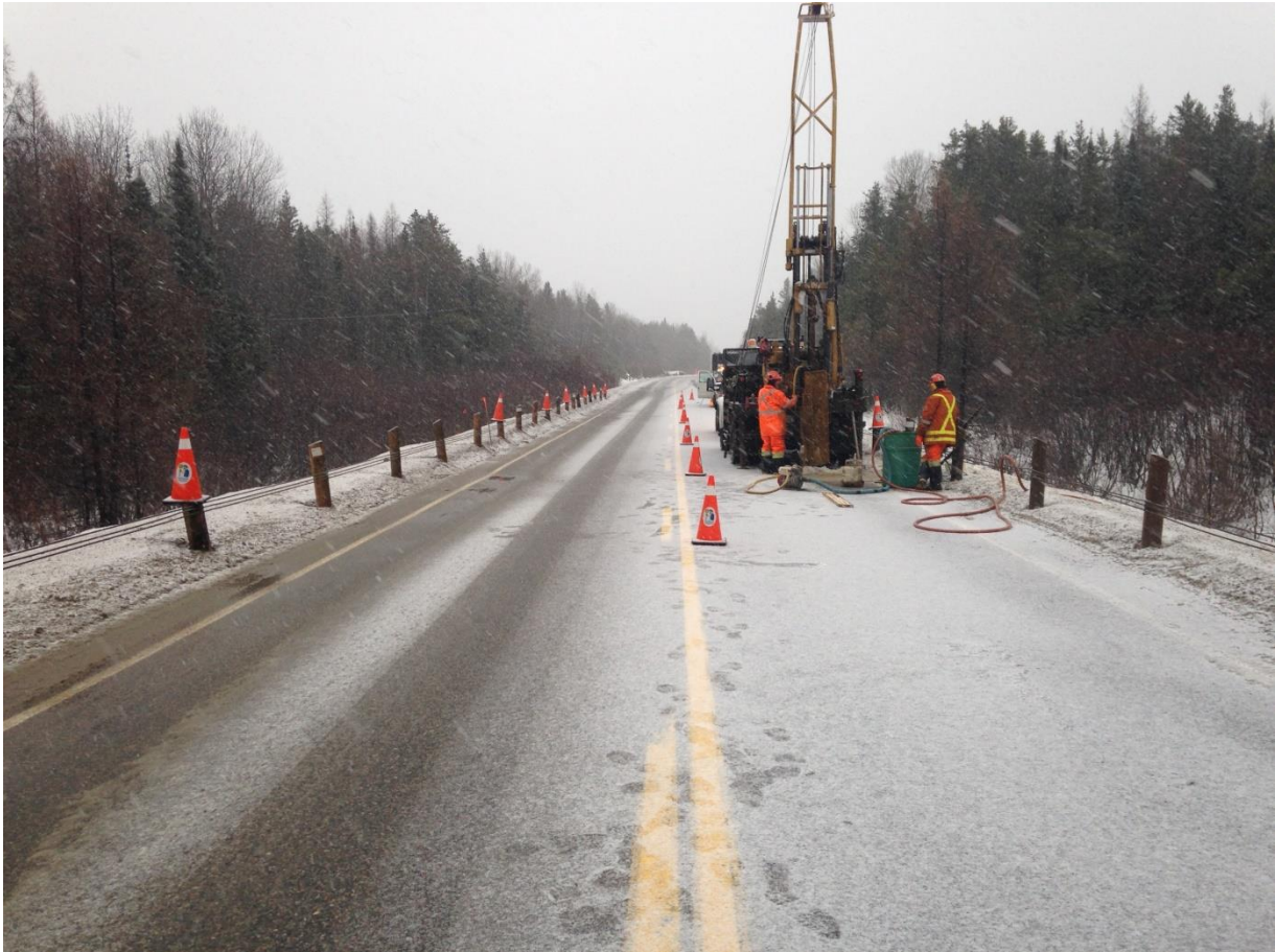
Photograph P1: Looking south at the location of Borehole PCN-2. The borehole drilled at Highway 129 SB shoulder. (December 16, 2014)
