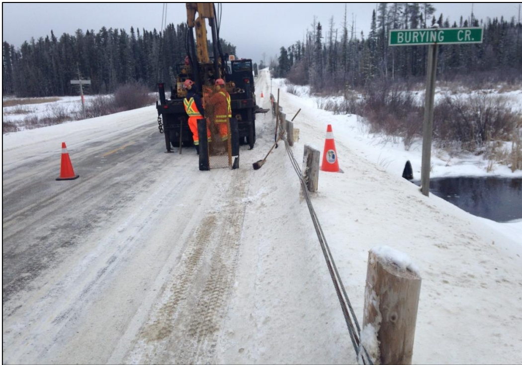
Photograph P3: Looking north from Highway 129 northbound lane shoulder. Borehole BC-3 advanced using a truck-mounted drill rig. (December 12, 2014)
