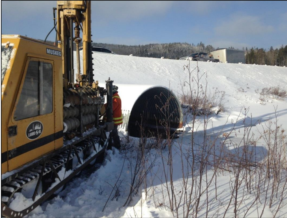
Photograph P1: Looking north at the location of Borehole SR-4. The inlet of the existing CSP culvert is visible. (January 12, 2015)
