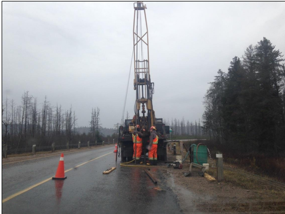
Photograph P4: Looking south from Highway 129 southbound lane shoulder. Borehole SR-5 advanced using a truck-mounted drill rig. (November 18, 2015)
