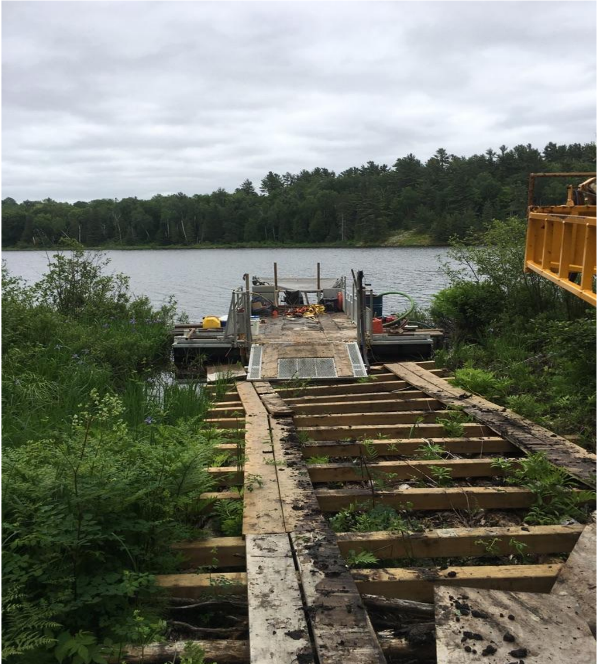
Photograph 2: The barge launching deck was built at site to facilitate access for barge and drill rig (May 2017).
