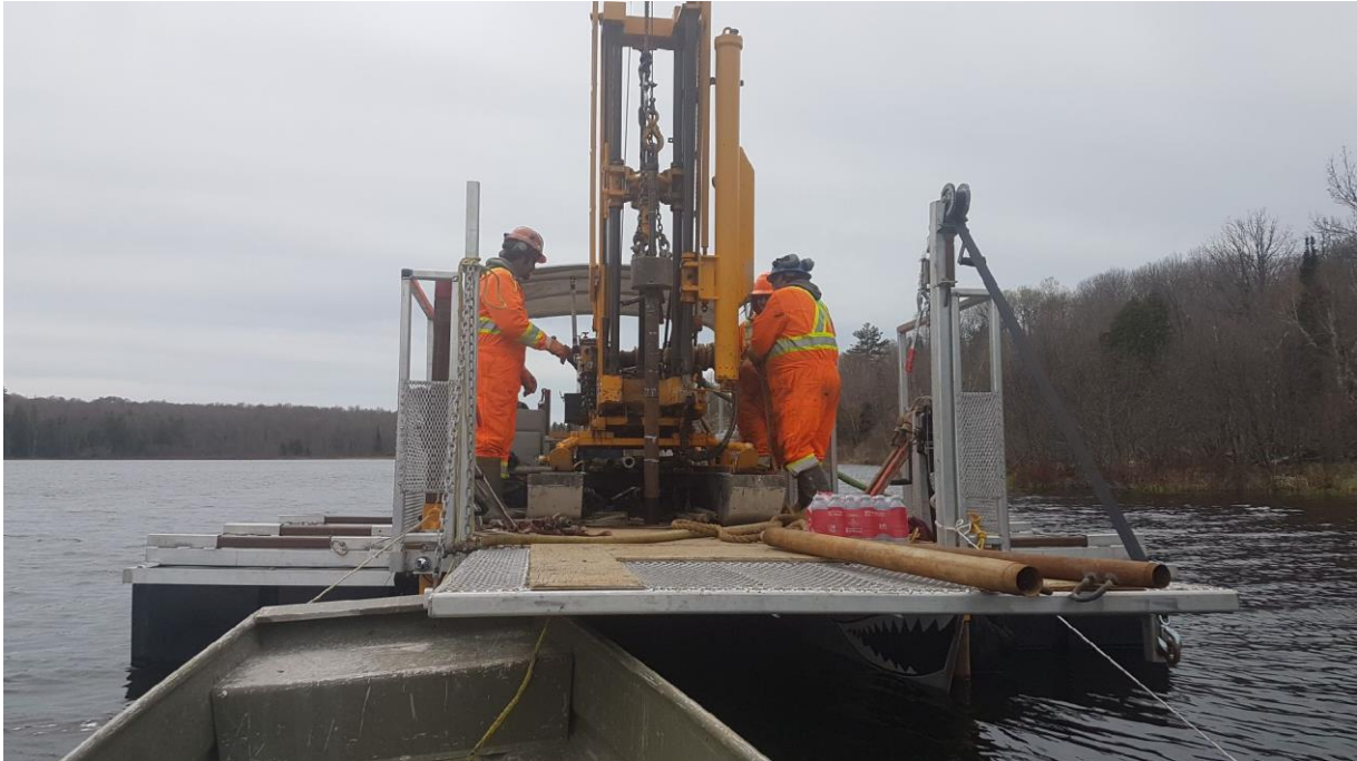
Photograph 3: The Skid Mounted Diedrich D-25 drill rig loaded on barge to mobilize drill rig to borehole locations (June 2017).
