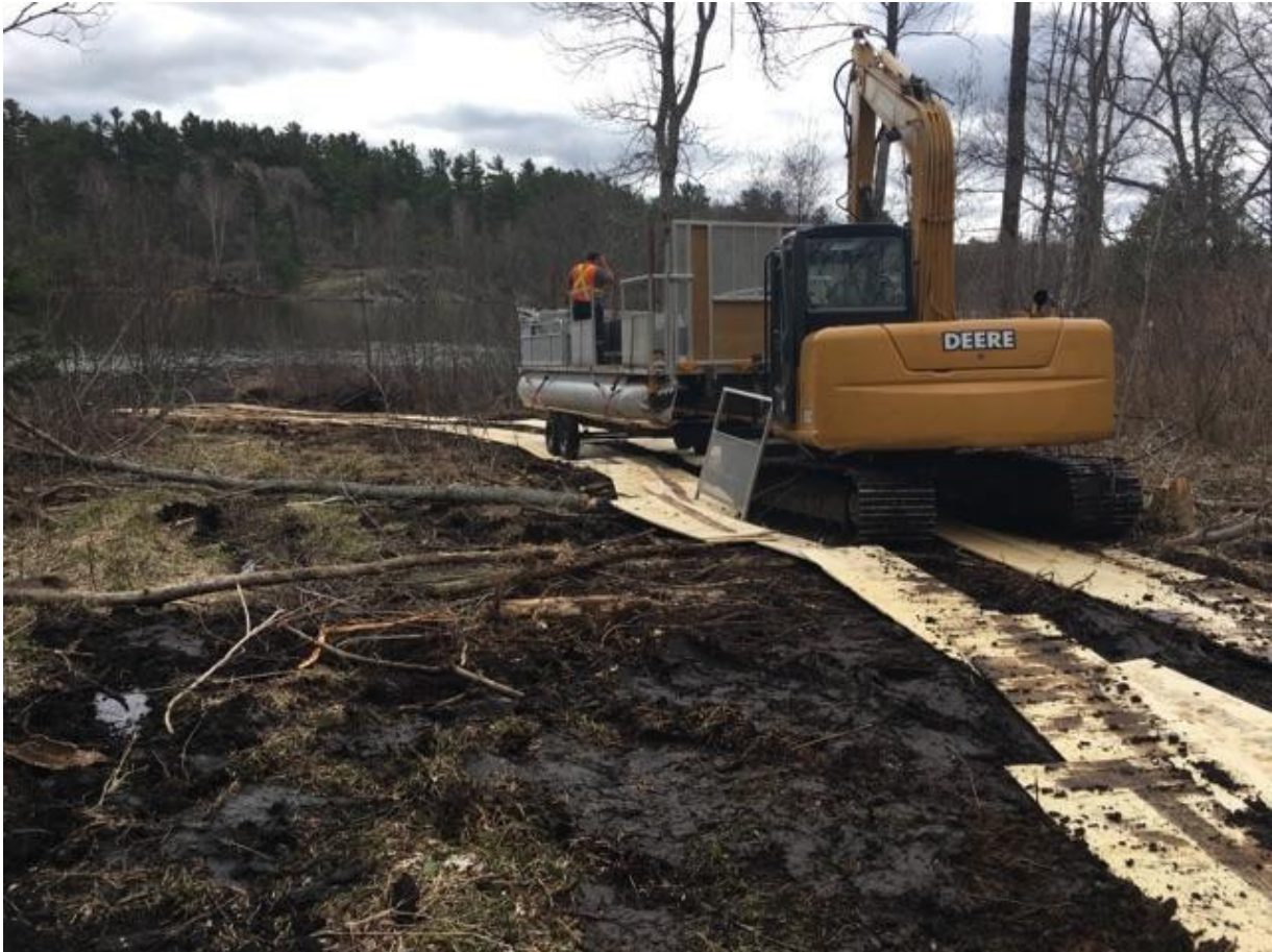
Photograph 1: Due to soft and swampy condition of the access route, plywood was used to facilitate access to the lake (May 2017).
