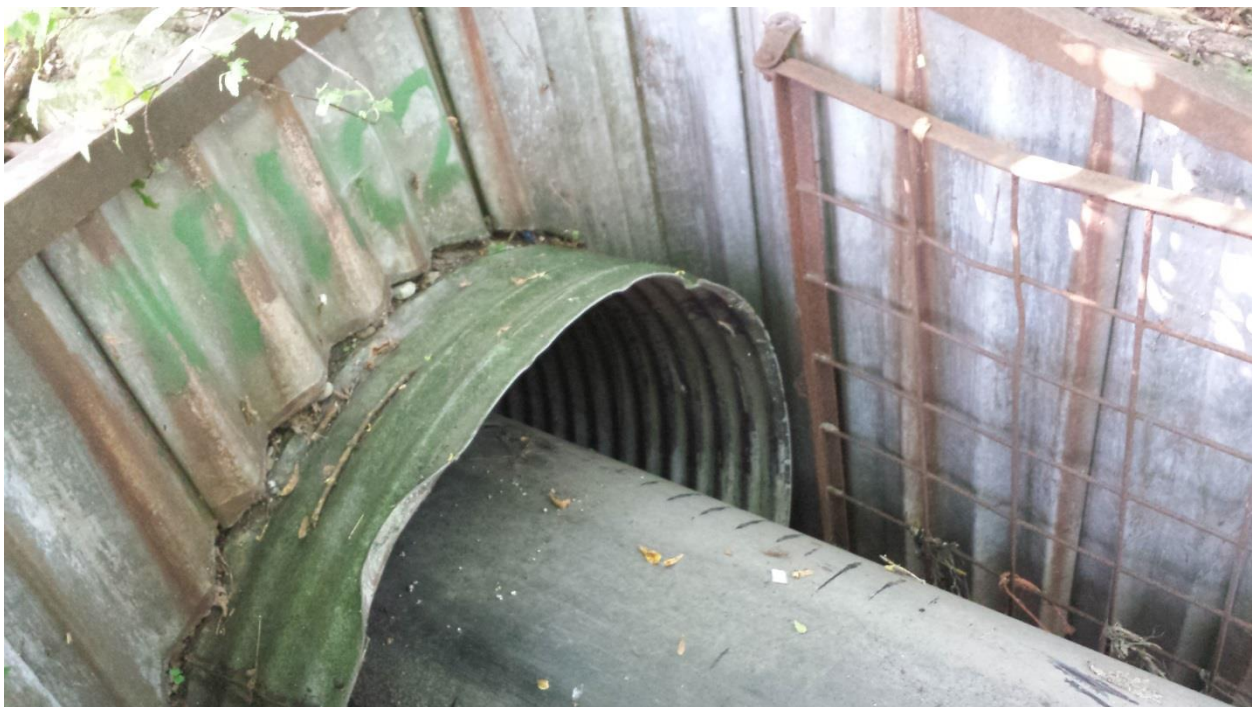
Photograph P2: Looking at the pipe outlet. The CSP pipe and HDPE liner are visible. The HDPE liner sheared off and slipped down the slope to the Don River (August 8, 2014).
