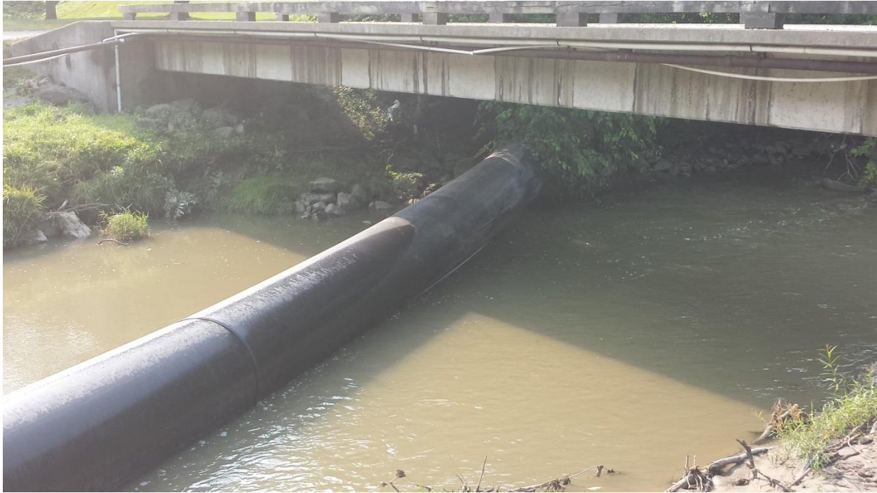
Photograph P3: Looking north at the location of the pipe outlet. The HDPE liner slipped down the slope to the Don River (August 8, 2014).
