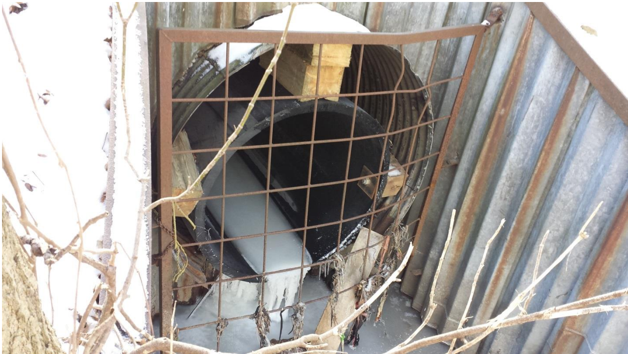
Photograph P5: Looking at the pipe outlet. The HDPE liner is cut off and temporary braced with blocks and bolts at the outlet (January 14, 2015).
