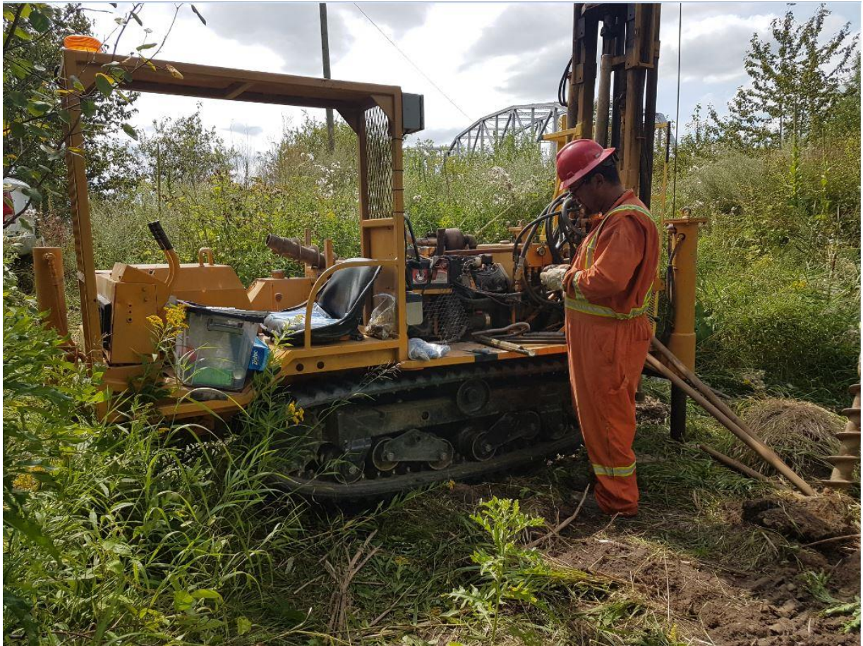
Photograph 6 – Drilling Setup of Borehole 16-5, Toe of the Approach Embankment (August 10, 2016).
