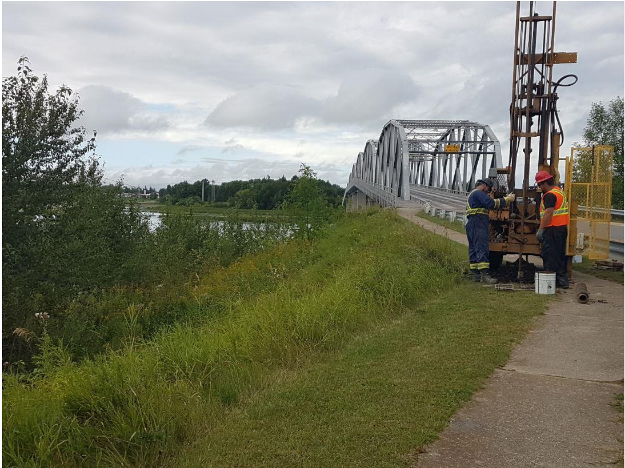
Photograph P4 – Looking West at Drilling of Borehole 16-4, Located at the top of the Approach Embankment (August 11, 2016).
