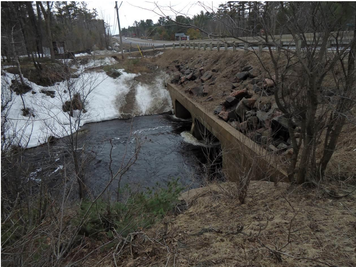
Photograph 3: Upstream Wall, looking south. Note the obvert of the culvert to be higher than the outlet in Photograph 2. (Photograph taken on April 14, 2014)
