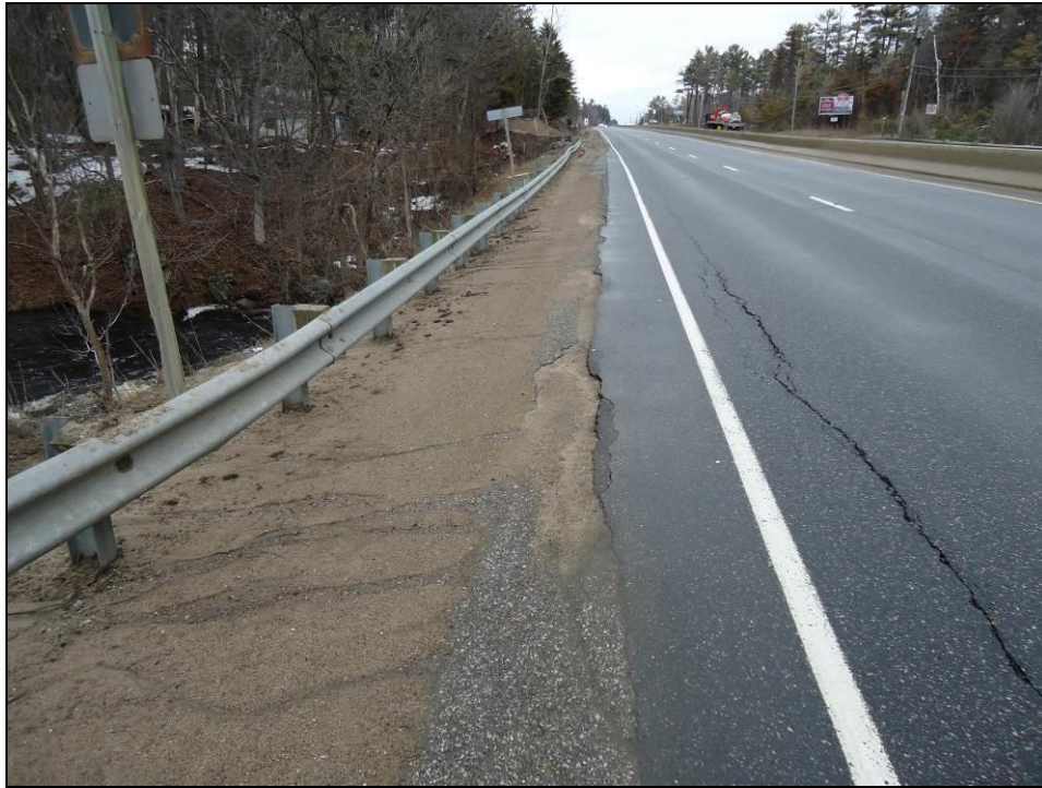
Photograph 1: Taken from the Highway 11 southbound lane outside shoulder, south of the Kahshe River looking north. Note the longitudinal crack approximately 0.3 m east of the Highway 11 southbound lane shoulder. (Photograph taken on April 14, 2014)
