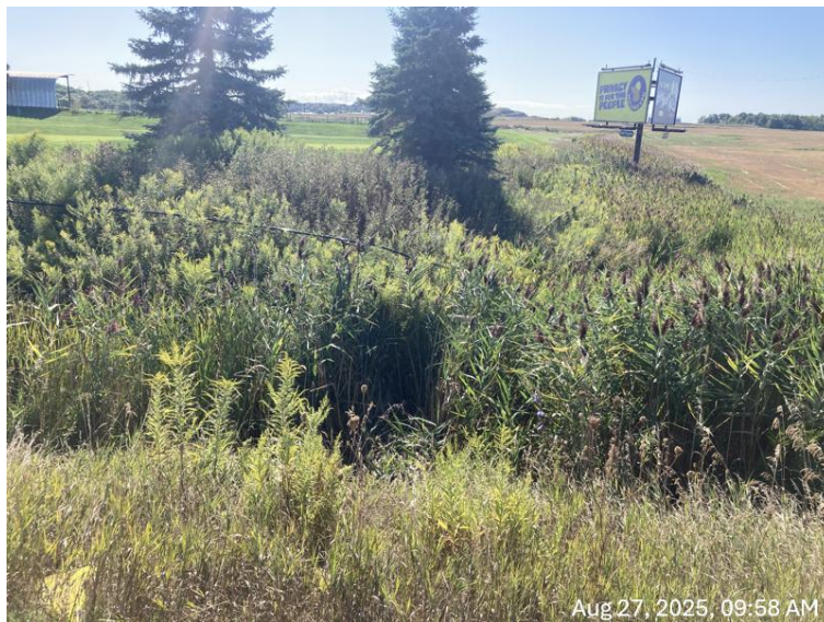
Figure 1: Proposed Culvert Extension Location (Looking South)
