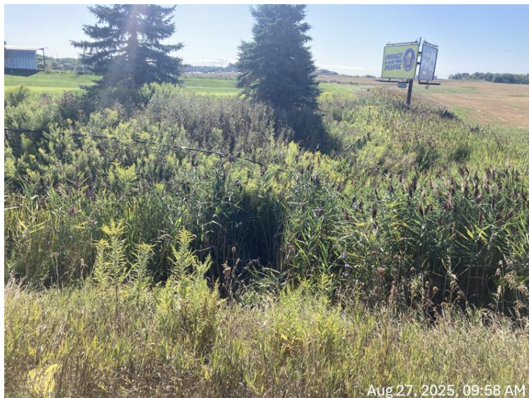
Figure 1: Proposed Culvert Extension Location (Looking South)
