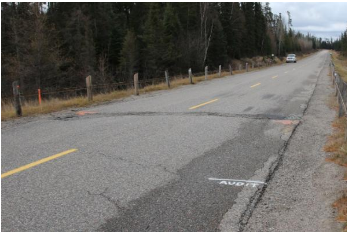
Photograph No. 2 – Pavement Cracking at Culvert (Facing South)
