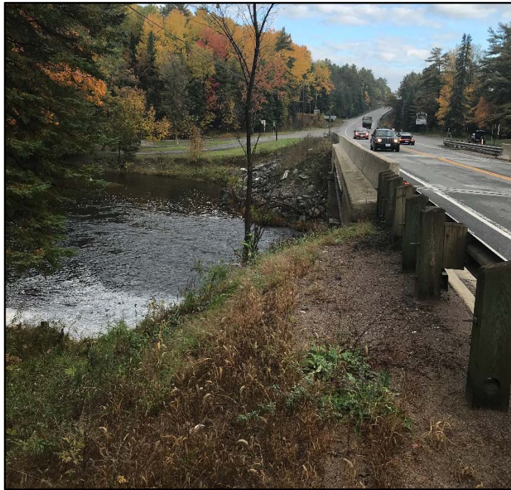
Photograph 5 – West side of Highway 28 looking north. Rock fill observed on surface of northwest approach embankment side slope.
