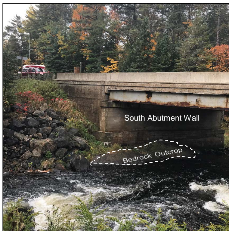
Photograph 4 – South abutment and bedrock outcrop – looking southwest from north side of creek
