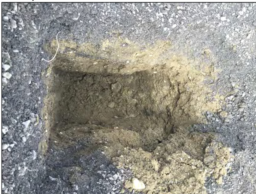
Photo B-12: Open TP15-06 showing Granular A and B fill and sandy silt (fill) materials used to cover north TDA area.
