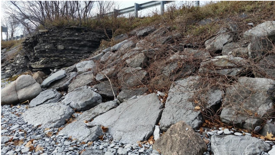
Plate 3: Typical Stone Revetment in Place along Highway 33
