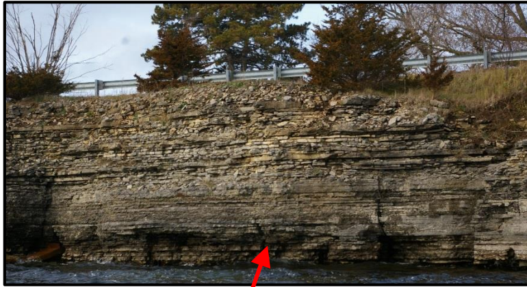
Differential Weathering of the Rock Face Resulting in Overhangs
