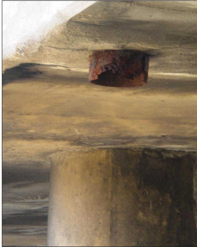
Photograph 25: Rusted Deck Drain.
