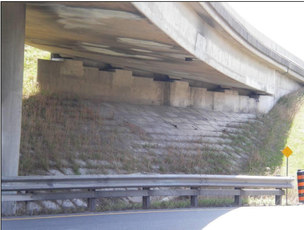
Photograph 10: South Slope Paving.
