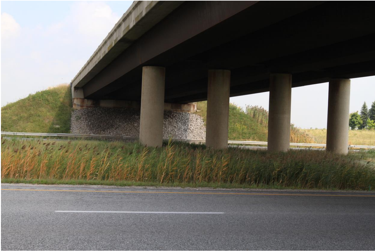
Photograph 3: Central Pier Supports seem to be in good condition with no cracking observed on piers (September 2, 2015).
