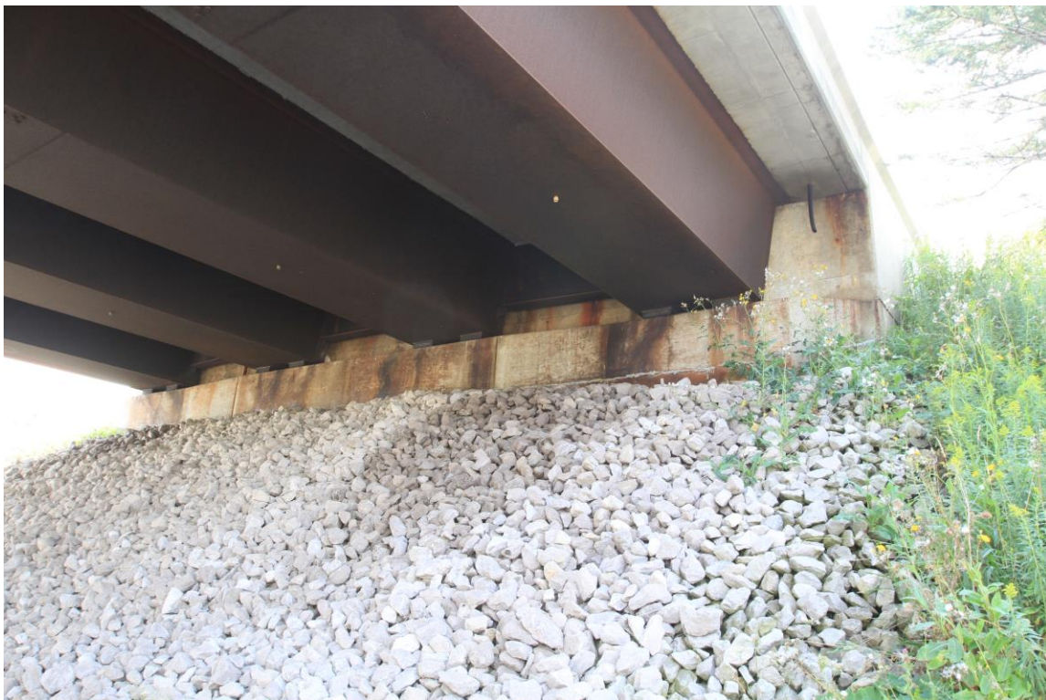
Photograph 2: South Abutment and East Wingwall of East Bound Lane. Central portion of abutment covered with rip rap (September 2, 2015).
