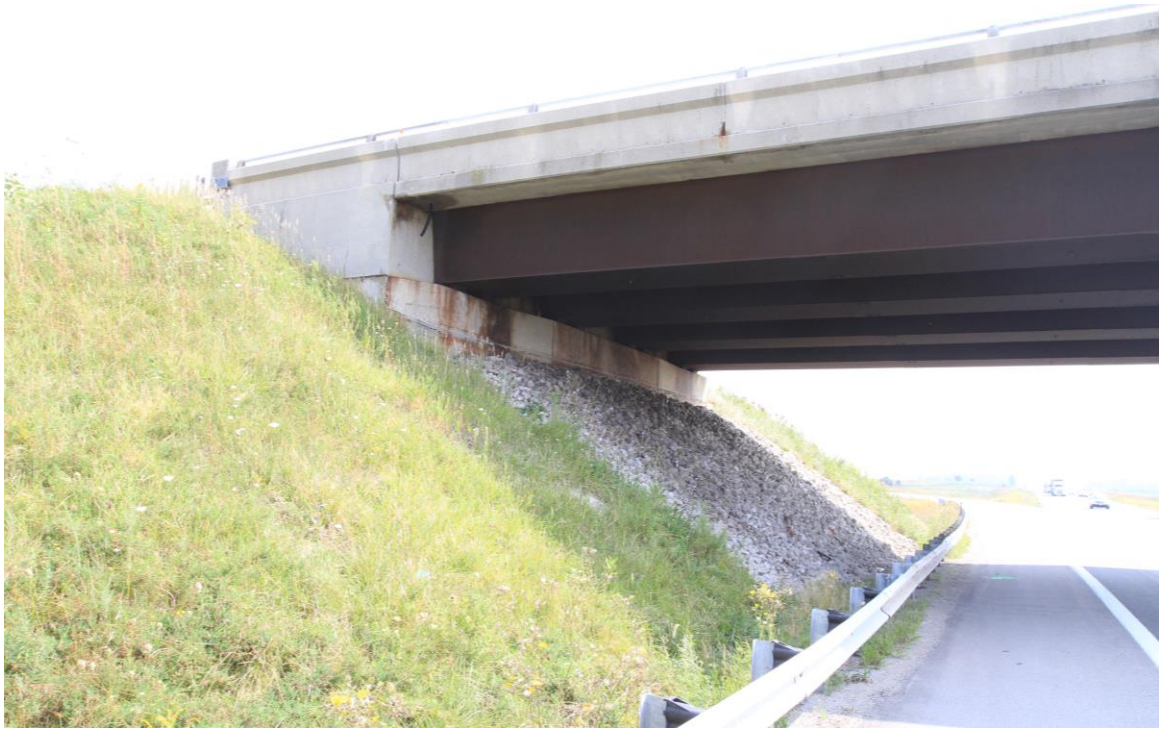
Photograph 1: North Abutment and West Wingwall of West Bound Lane. Abutment slopes are grass covered and no obvious signs of erosion observed on slope. Central portion covered with rip rap (September 2, 2015).
