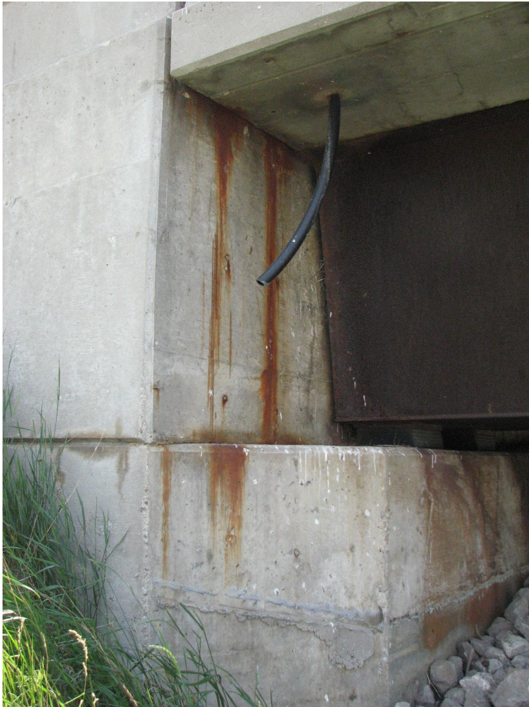
Photograph 4: South Abutment and East Wingwall. No obvious signs of cracking observed on the wall (September 2, 2015).
