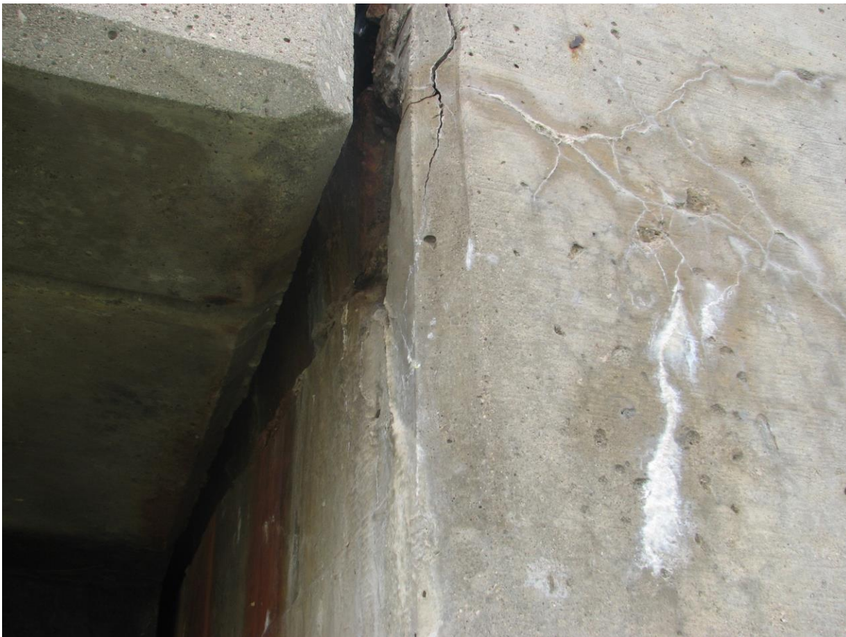
Photograph 5: North Abutment and East Wingwall. Minor cracks observed on this wall (September 2, 2015).
