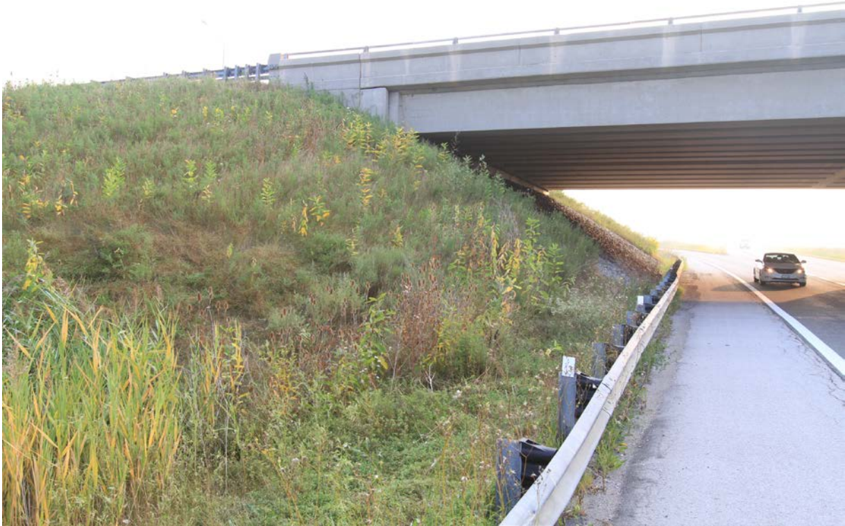
Photograph 2: Looking at the west wingwall and the adjacent slope of north abutment of the Colonel Talbot Road (Highway 4) Underpass Structure from Highway 402. Surficial cracks were observed on the wingwall. The slope is vegetated and effect of erosion on the slope face was not observed (September 2, 2015).
