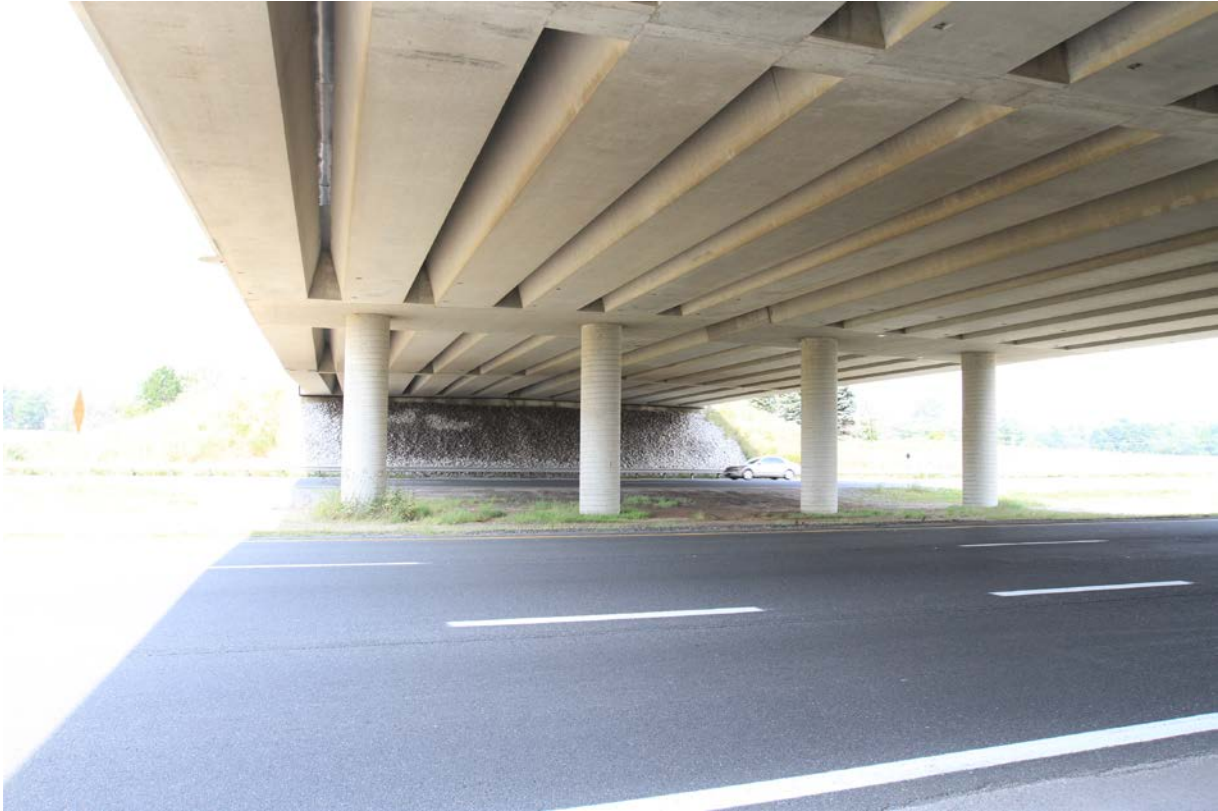
Photograph 8: Looking at the center piers at the south shoulder of EBL of Highway 402. Surficial cracks were observed on the piers. The ground around the piers was partially covered with vegetation and the effect of erosion on the ground surface was not observed (September 2, 2015).
