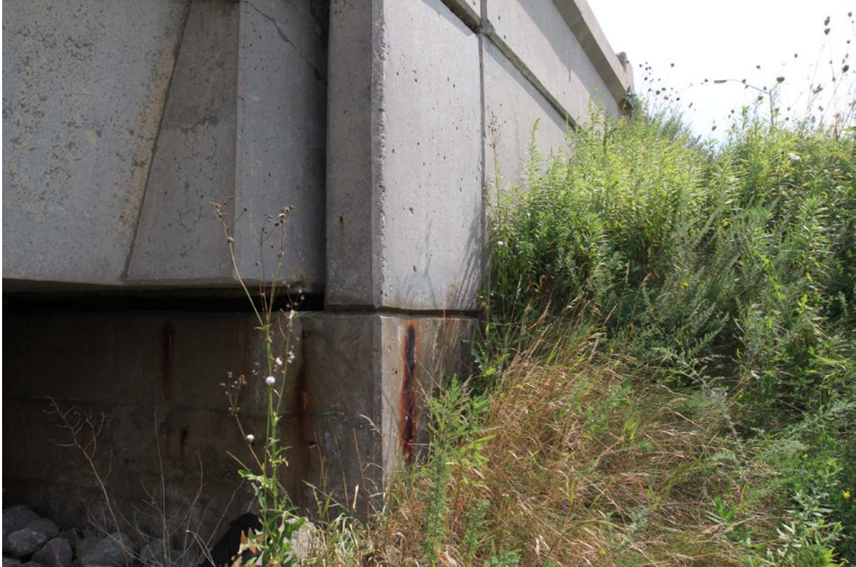
Photograph 5: Looking at the south abutment wall, west wingwall and the adjacent slope of the south abutment of the Colonel Talbot Road (Highway 4) Underpass Structure from Highway 402. Surficial cracks were observed on the abutment wall and wingwall. The slope is vegetated and effect of erosion on the slope face was not observed (September 2, 2015).
