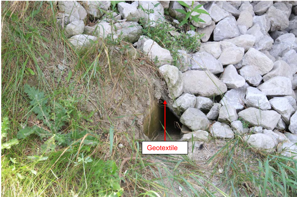
Photograph 7: Looking at the void at the south abutment. A concrete element was exposed (September 2, 2015).
