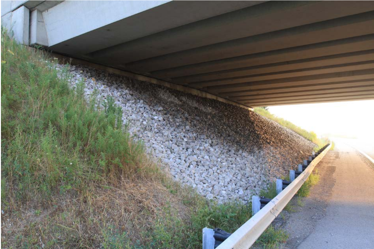
Photograph 1: Looking at the north abutment of the Colonel Talbot Road (Highway 4) Underpass Structure from Highway 402. Surficial cracks were observed on the abutment wall. Rock protection is provided on the front slope of the abutment. Effect of erosion on the slope face was not observed on the slope face (September 2, 2015).
