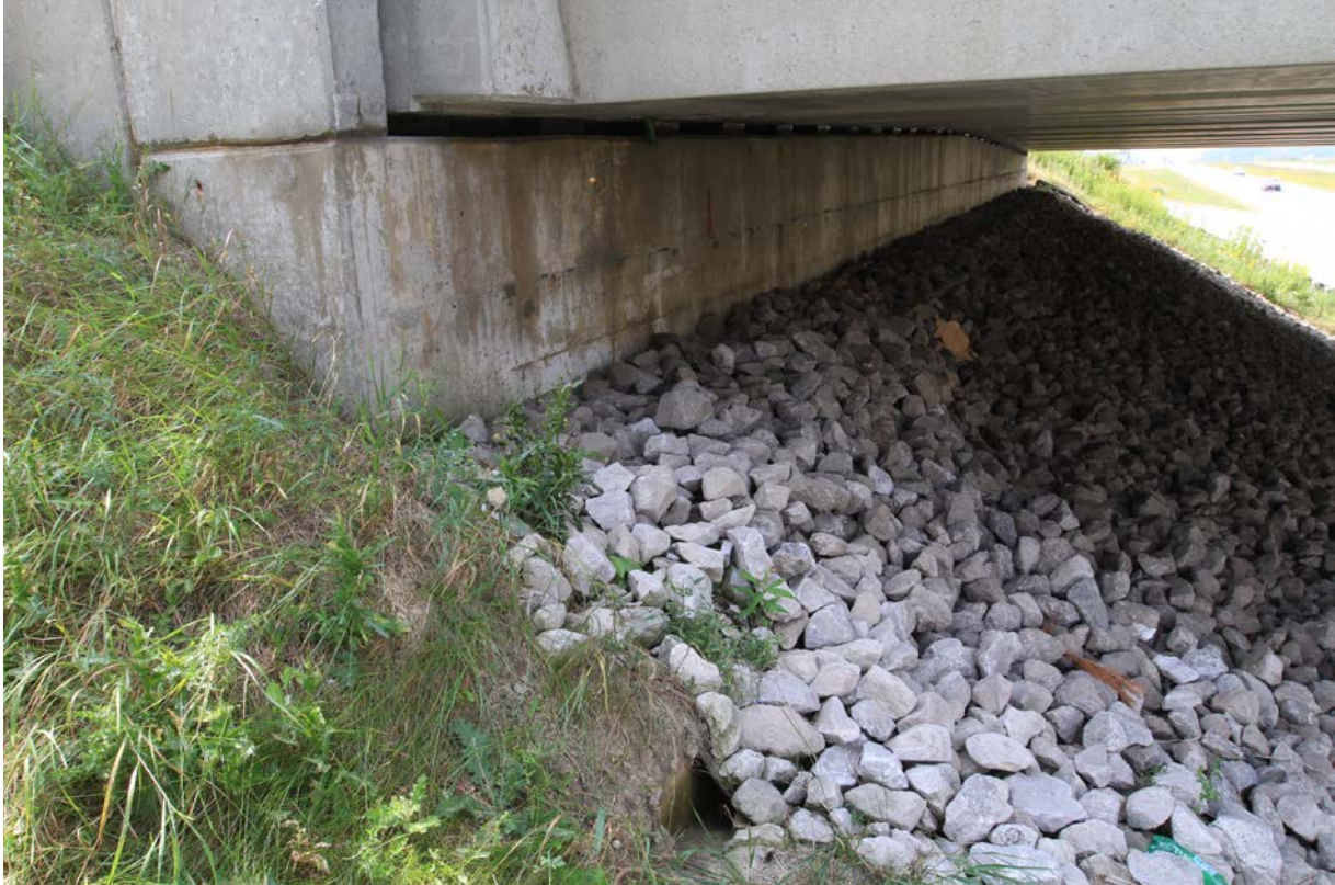
Photograph 6: Looking at the south abutment, east wingwall and the adjacent slope of the south abutment of the Colonel Talbot Road (Highway 4) Underpass Structure from Highway 402. Surficial cracks were observed on the abutment and wingwalls. Rock protection is provided on the front slope of the abutment. A void was observed underneath the rock protection. The adjacent slope is vegetated and effect of erosion on the slope face was not observed (September 2, 2015).
