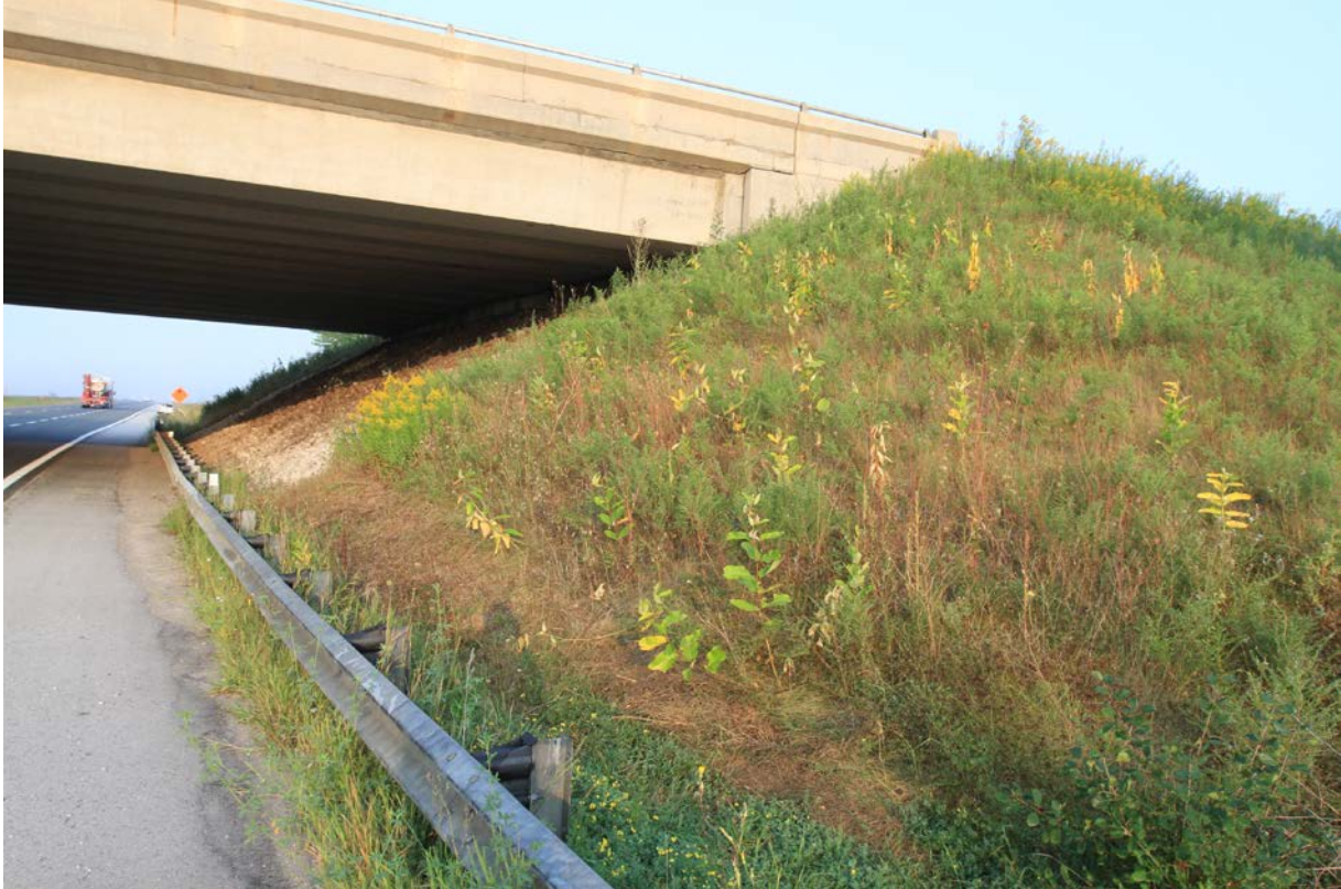
Photograph 3: Looking at east wingwall and the adjacent slope of north abutment of the Colonel Talbot Road (Highway 4) Underpass Structure from Highway 402. Surficial cracks were observed on the wingwall. The slope is vegetated and effect of erosion on the slope face was not observed (September 2, 2015).
