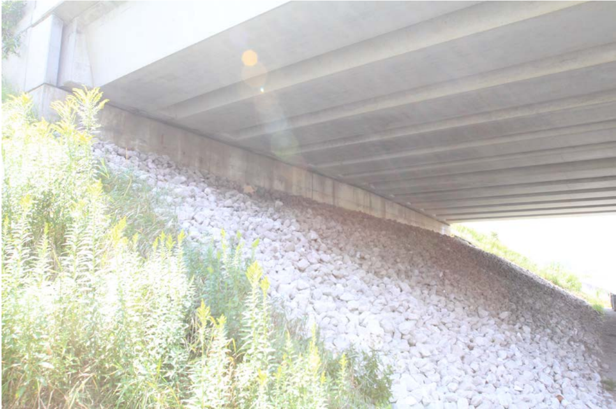
Photograph 4: Looking at the south abutment of the Colonel Talbot Road (Highway 4) Underpass Structure from Highway 402. Surficial cracks were observed on the abutment wall. Rock protection is provided on the front slope of the abutment. Effect of erosion on the slope face was not observed (September 2, 2015).
