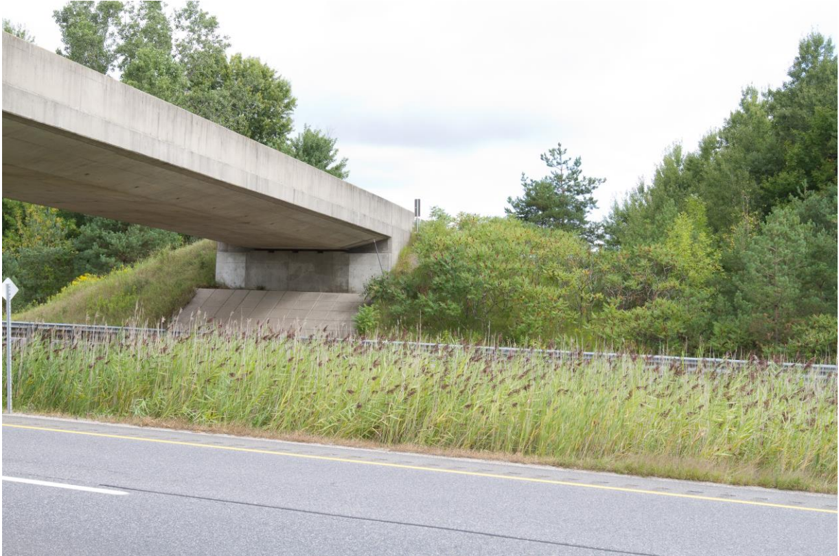
Photograph 7: Looking at the east wingwall and the adjacent slope of the north abutment of the West Quarter Townline Road Underpass Structure. Minor cracks were observed on the wingwall. The slope is vegetated and erosion on the slope face was not observed (August 28, 2015).
