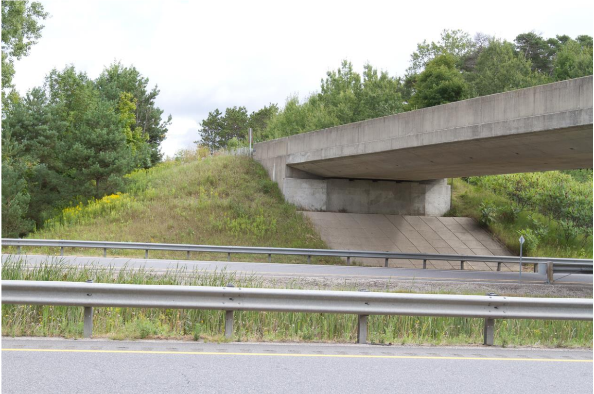
Photograph 6: Looking at the west wingwall and the adjacent slope of the north abutment of the West Quarter Townline Road Underpass Structure. Surficial cracks were observed on the wingwall. The slope is vegetated and erosion on the slope face was not observed (August 28, 2015).
