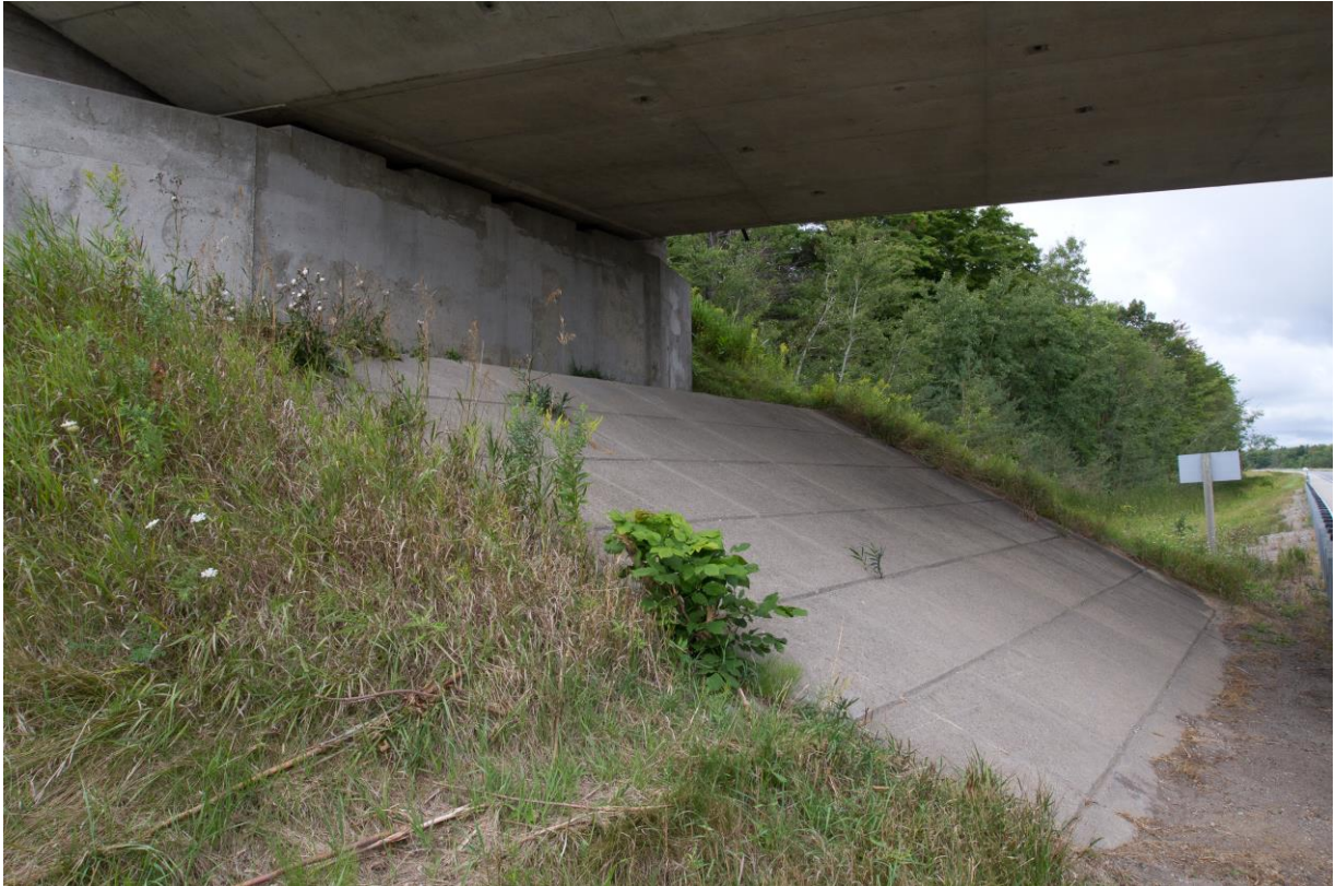
Photograph 1: Looking at the south abutment of the West Quarter Townline Road Underpass Structure. Vertical cracks were observed on the abutment wall. Weep holes were not observed in the abutment wall. Sealant between the concrete panels appeared degraded at locations where grasses and shrubs are growing. The toe of the front slope was covered with soil (August 28, 2015).
