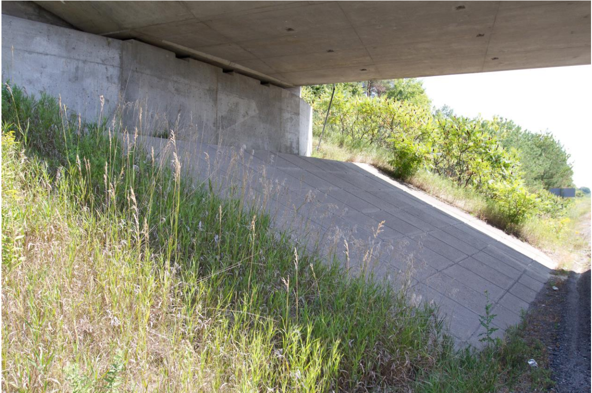
Photograph 2: Looking at the north abutment of the West Quarter Townline Road Underpass Structure. Vertical cracks were observed on the abutment wall. Sealant between the concrete panels appeared degraded at locations. Weep holes were not observed in the abutment wall. The toe of the front slope was covered with soil (August 28, 2015).
