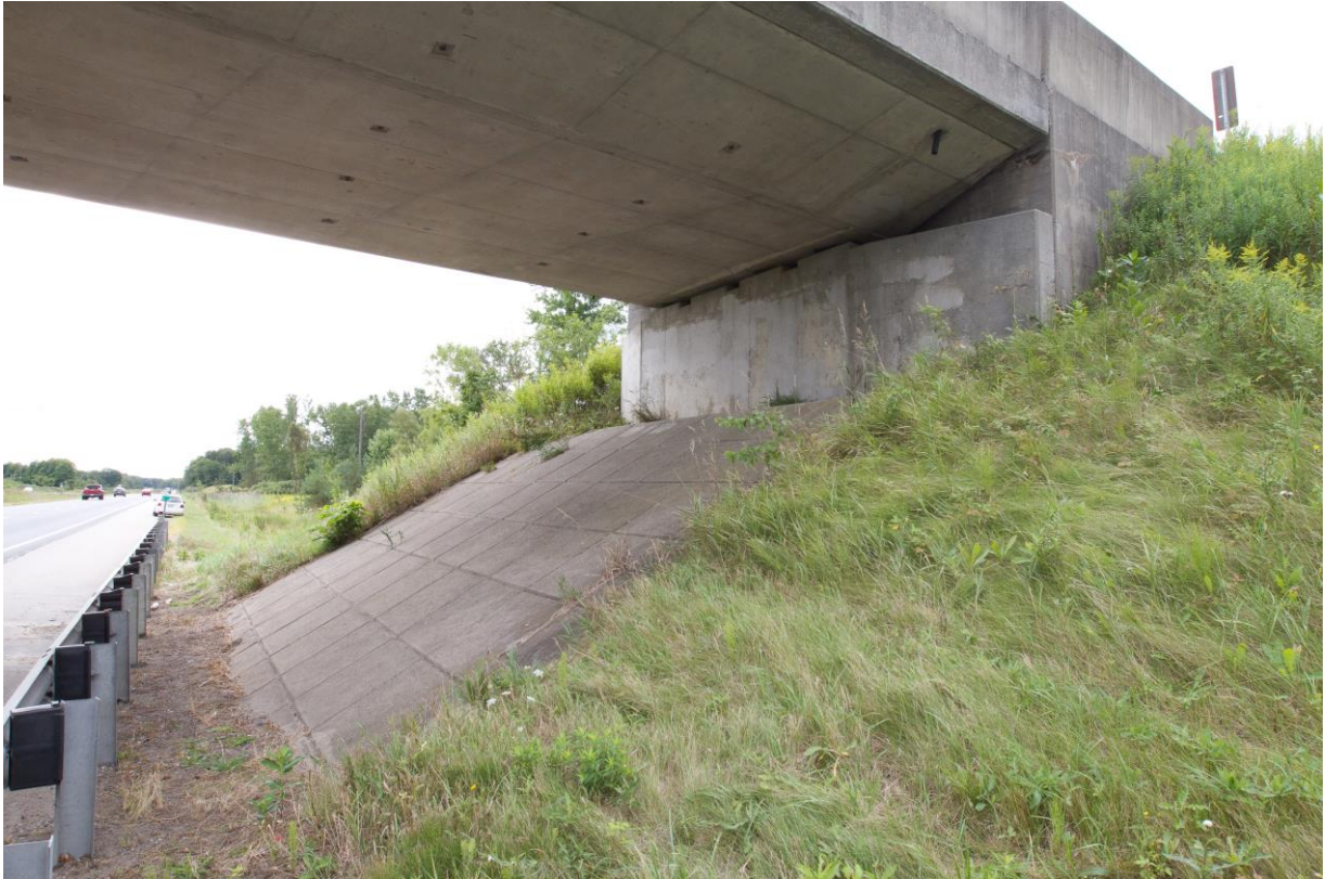
Photograph 5: Looking at the west wingwall and the adjacent slope of the south abutment of the West Quarter Townline Road Underpass Structure. Surficial cracks were observed on the wingwall. The slope is vegetated and erosion on the slope face was not observed (August 28, 2015).
