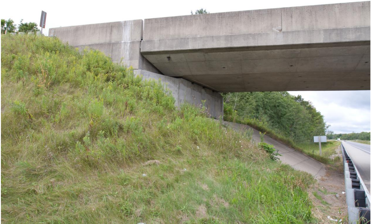
Photograph 4: Looking at the east wingwall and the adjacent slope of the south abutment of the West Quarter Townline Road Underpass Structure. Surficial cracks were observed on the wingwall. The slope is vegetated and erosion on the slope face was not observed (August 28, 2015).
