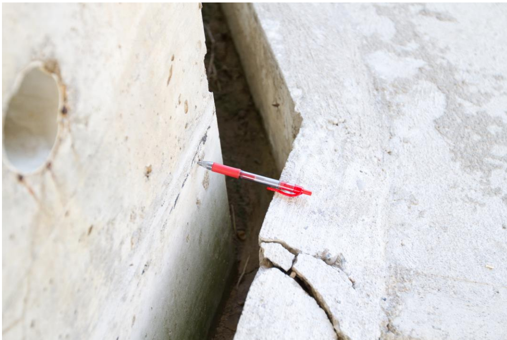
Photograph 3: Looking at the gap between the abutment wall and concrete panel (August 28, 2015).
