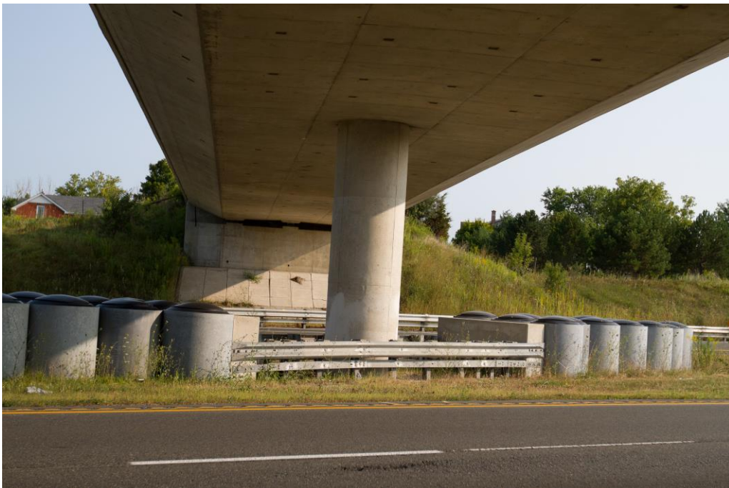
Photograph 7: Looking north at the pier of Jerseyville Road Underpass Structure. Surficial cracks were observed on the pier (August 28, 2015).
