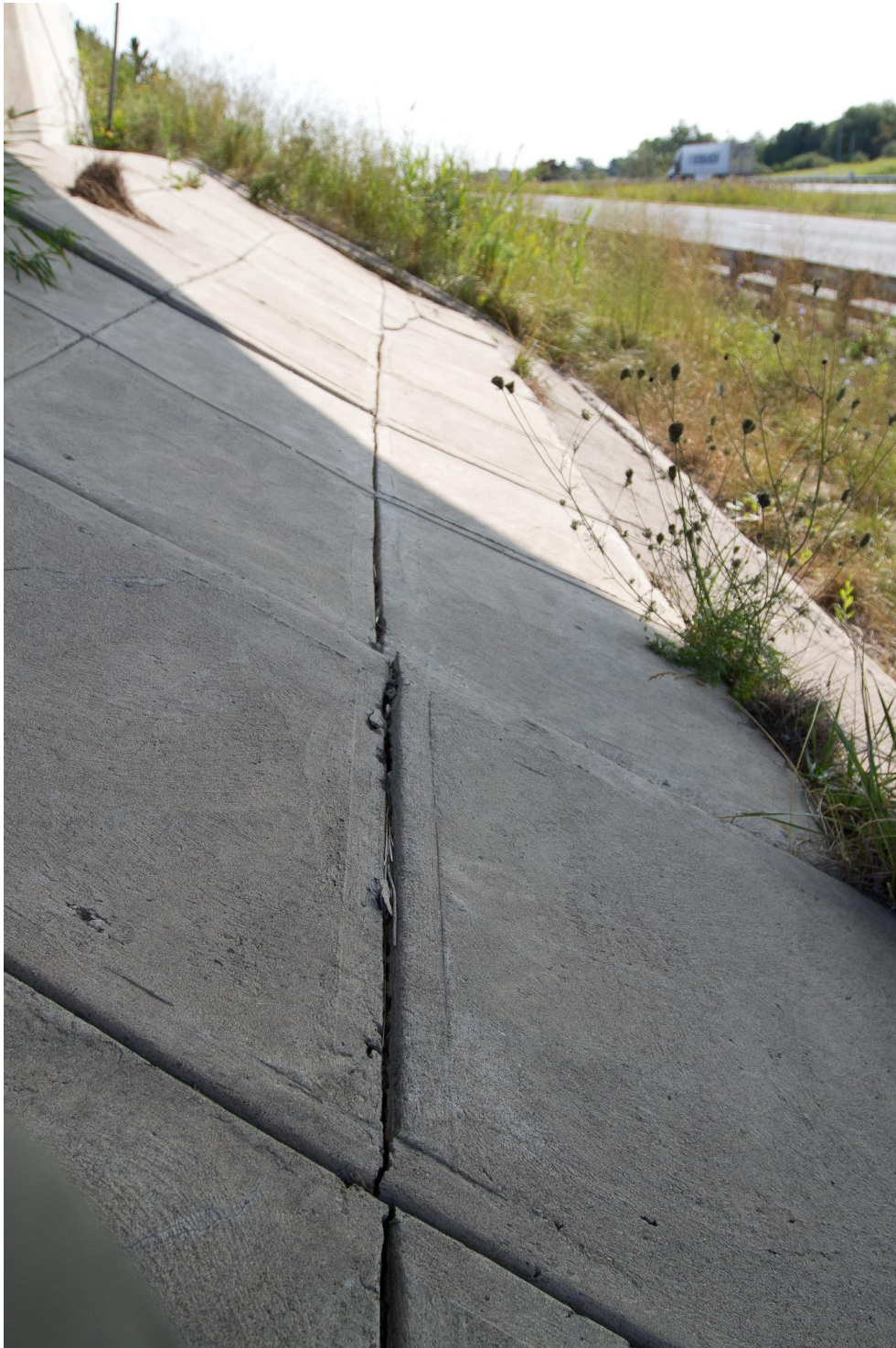
Photograph 5: Looking at the concrete panels on the front slope of the north abutment. Cracks and dislodge of concrete panels observed (August 28, 2015).
