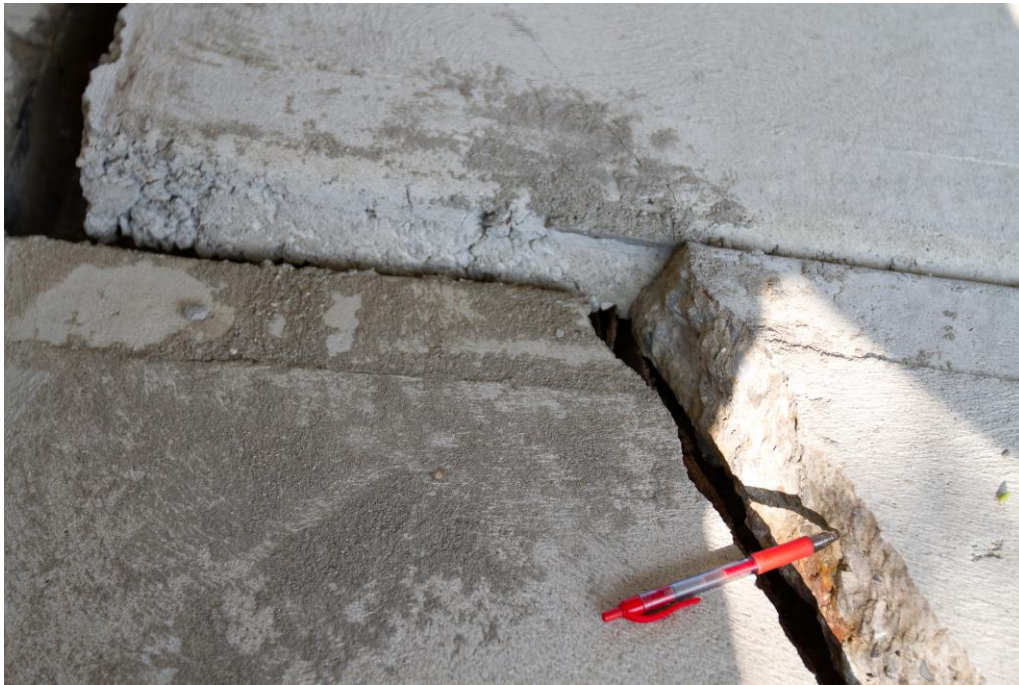
Photograph 2: Looking at the concrete panels on the front slope of the south abutment. Breaks and dislodge of concrete panels observed (August 28, 2015).
