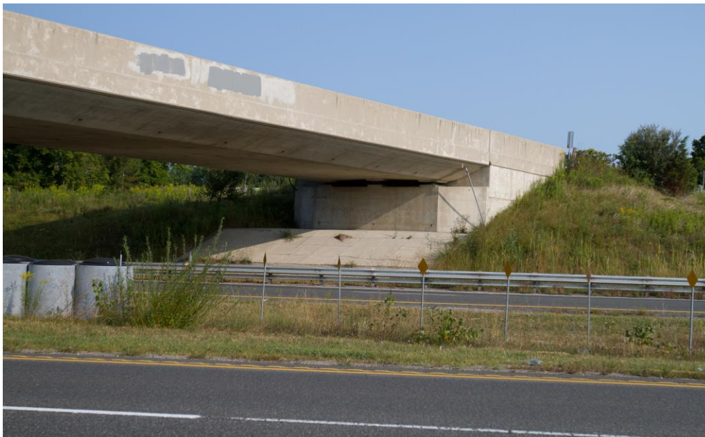
Photograph 11: Looking at the east wingwall and the adjacent slope of the north abutment of the Jerseyville Road Underpass Structure. Minor cracks were observed on the wingwall. The slope is vegetated and effect of erosion on the slope face was not observed (August 28, 2015).
