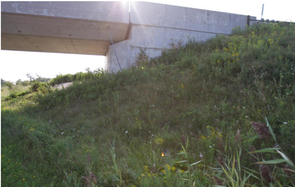
Photograph 9: Looking at the west wingwall and the adjacent slope of the south abutment of the Jerseyville Road Underpass Structure. Surficial cracks were observed on the wingwall. The slope is vegetated and effect of erosion on the slope face was not observed (August 28, 2015).
