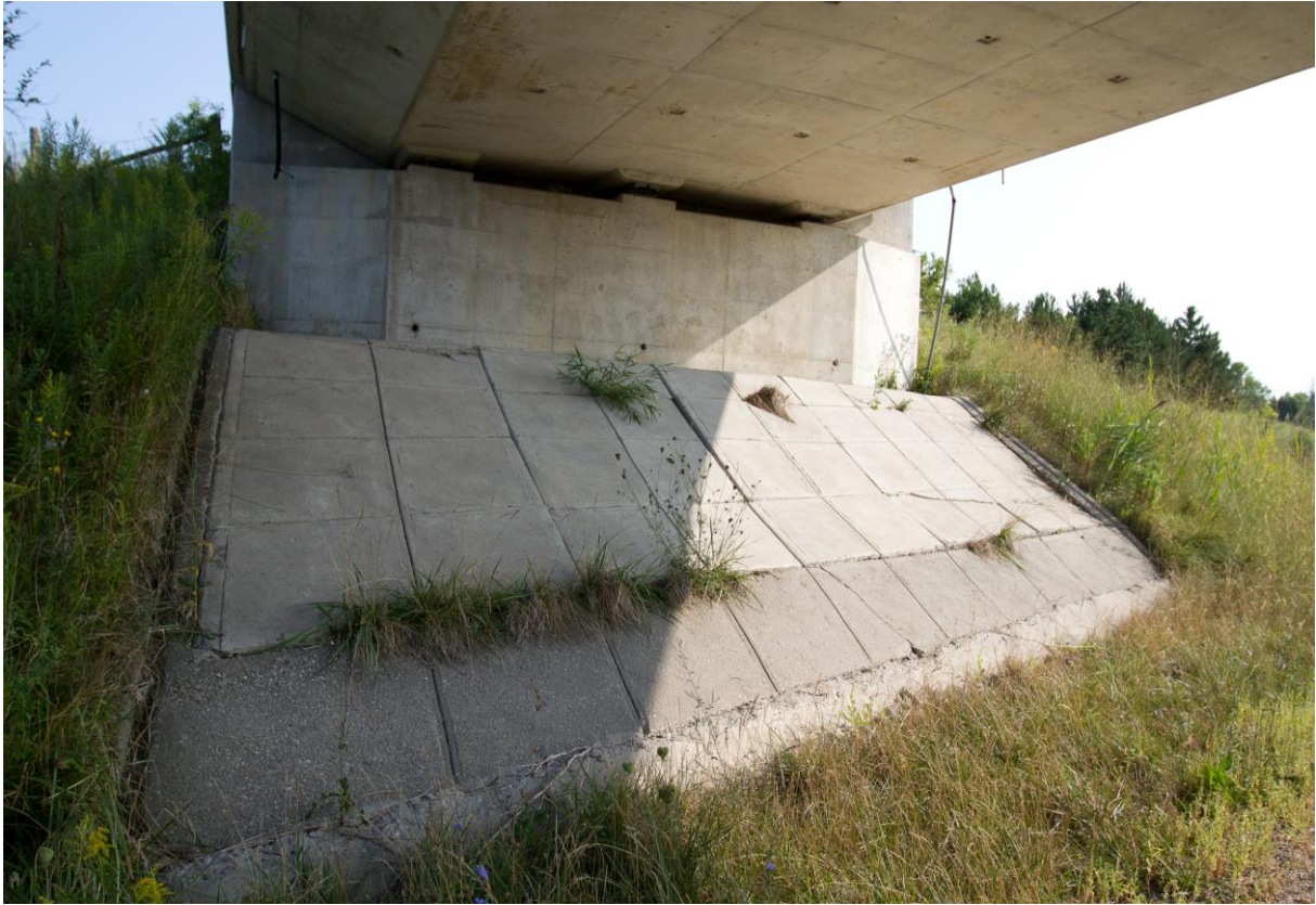
Photograph 4: Looking at the north abutment of the Jerseyville Road Underpass Structure. Vertical cracks were observed on the abutment wall. Weep holes were observed in the abutment wall. Sealant between the concrete panels appeared degraded at locations where grasses and shrubs are growing. Sloughing of ground underneath the concrete panels was observed. Cracks, breaks and dislodge of the concrete panels were also observed. The toe of the front slope was covered with vegetation (August 28, 2015).
