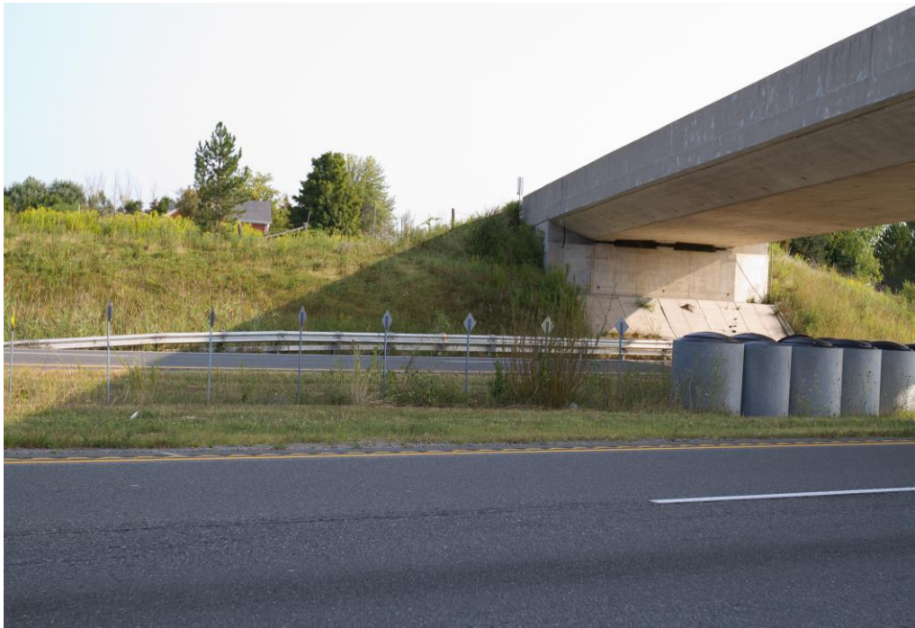
Photograph 10: Looking at the west wingwall and the adjacent slope of the north abutment of the Jerseyville Road Underpass Structure. Surficial cracks were observed on the wingwall. The slope is vegetated and effect of erosion on the slope face was not observed (August 28, 2015).
