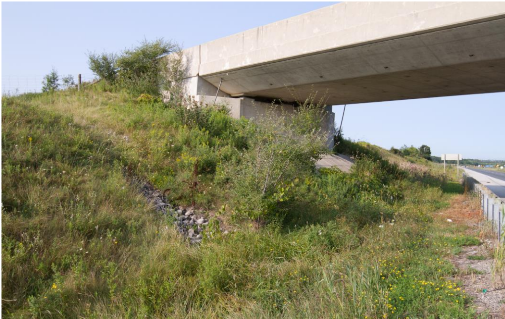
Photograph 8: Looking at the east wingwall and the adjacent slope of the south abutment of the Jerseyville Road Underpass Structure. Surficial cracks were observed on the wingwall. The slope is vegetated and effect of erosion on the slope face was not observed (August 28, 2015).
