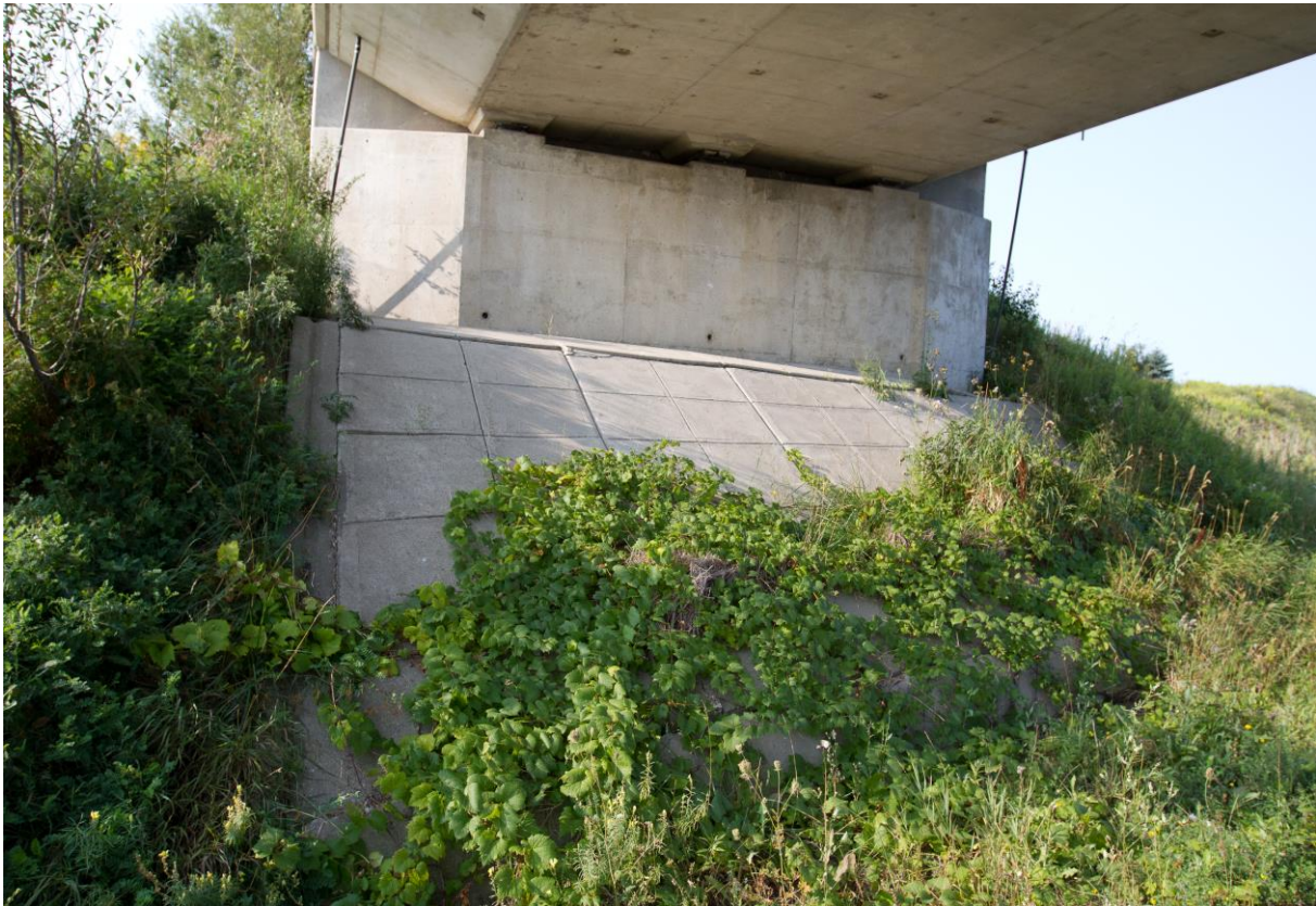
Photograph 1: Looking at the south abutment of the Jerseyville Road Underpass Structure. Vertical cracks were observed on the abutment wall. Weep holes were observed in the abutment wall. Sealant between the concrete panels appeared degraded at locations where grasses and shrubs are growing. Sloughing of ground underneath the concrete panels was observed. Cracks, breaks and dislodge of the concrete panels were also observed. The toe of the front slope was covered with vegetation (August 28, 2015).
