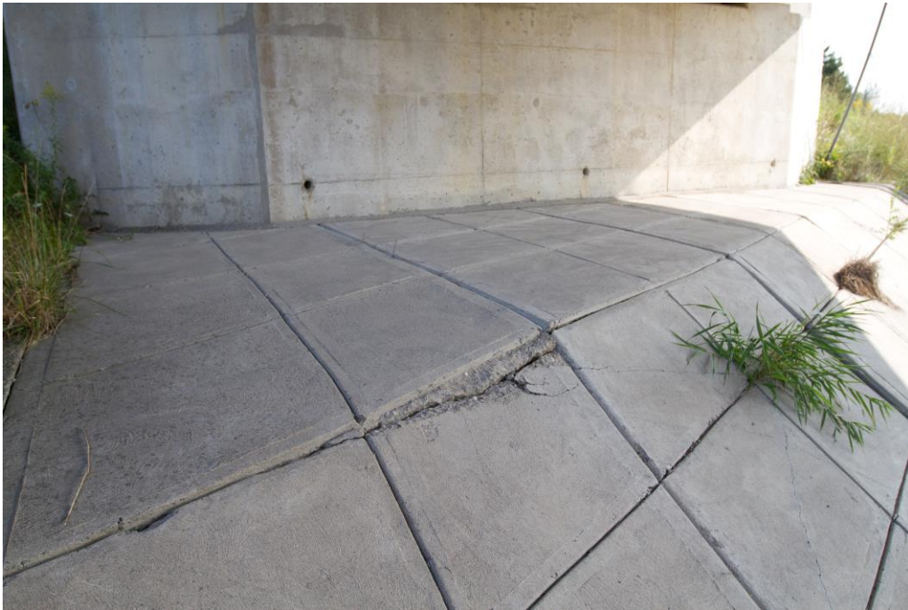
Photograph 6: Looking at the concrete panels on the front slope of the north abutment. Cracks on concrete panels observed (August 28, 2015).
