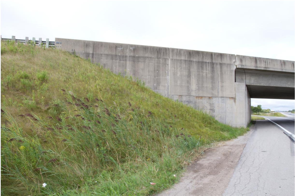
Photograph 2: Looking at the northeast wingwall and the adjacent slope of the east abutment of the Oxford Road 55 Underpass Structure. Surficial cracks were observed on the wingwall. The slope is vegetated and effect of erosion on the embankment slope face was not observed (August 28, 2015).
