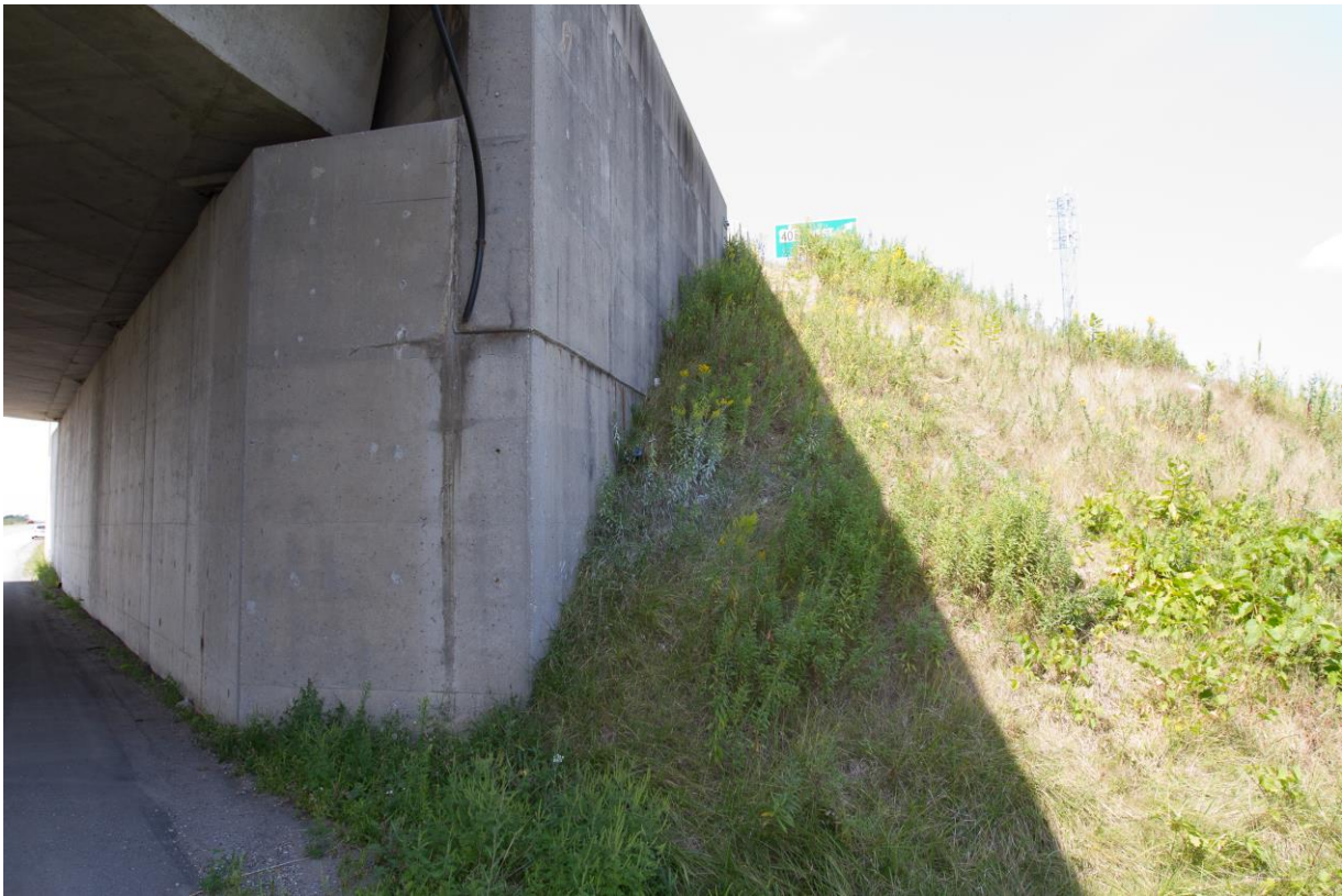
Photograph 5: Looking at the northwest wingwall and the adjacent slope of the west abutment of the Oxford Road 55 Underpass Structure. Cracks were observed on the wingwall. The slope is vegetated and effect of erosion on the slope face was not observed (August 28, 2015).
