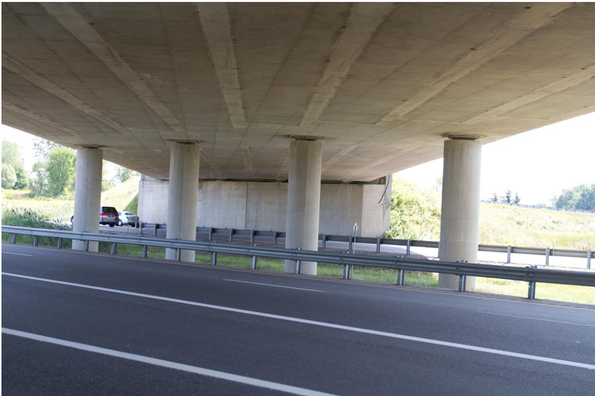
Photograph 7: Looking south at the piers of Oxford Road 55 Underpass Structure. Minor surficial cracks were observed on the piers (August 28, 2015).
