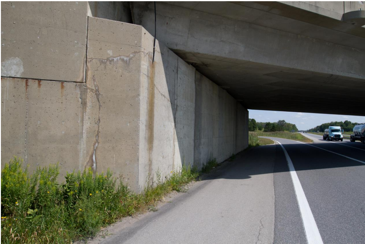
Photograph 4: Looking at the west abutment of the Oxford Road 55 Underpass structure. Vertical cracks were observed on the abutment wall. Horizontal and vertical cracks were observed on the southwest wingwall, where white salt staining was observed. Weep holes were observed in the abutment wall. Grasses are growing at the toe of abutment wall (August 28, 2015).
