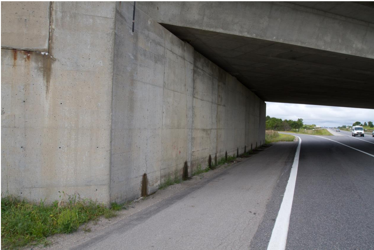
Photograph 1: Looking at the east abutment of the Oxford Road 55 Underpass structure. Vertical cracks were observed on the abutment wall. Weep holes were observed in the abutment wall. Grasses are growing at the toe of abutment wall (August 28, 2015).
