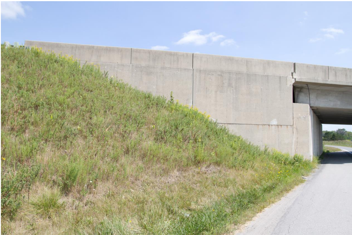
Photograph 6: Looking at the southwest wingwall and the adjacent slope of the west abutment of the Oxford Road 55 Underpass Structure. Surficial cracks were observed on the wingwall. The slope is vegetated and effect of erosion on the slope face was not observed (August 28, 2015).
