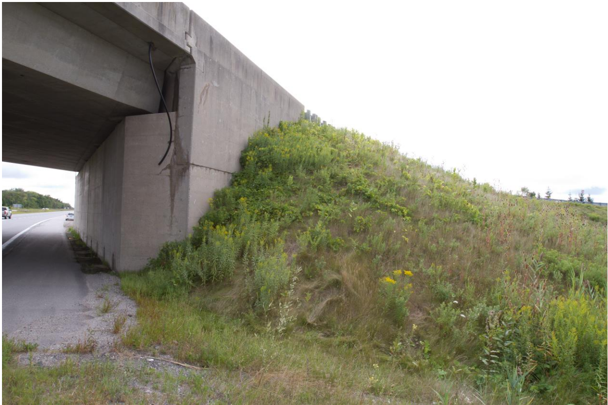
Photograph 3: Looking at the southeast wingwall and the adjacent slope of the east abutment of the Oxford Road 55 Underpass Structure. Surficial cracks were observed on the wingwall. Light spalling of concrete was observed at the joint of abutment wall and wingwall. The slope is vegetated and effect of erosion on the embankment slope face was not observed (August 28, 2015).
